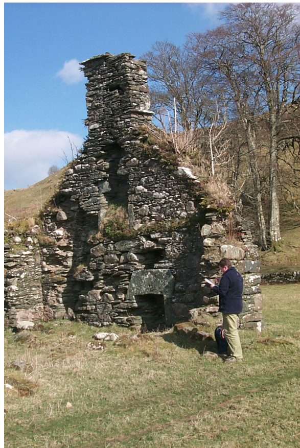
Figure 5.3 Glennan, north facing gable with integral fireplaces
