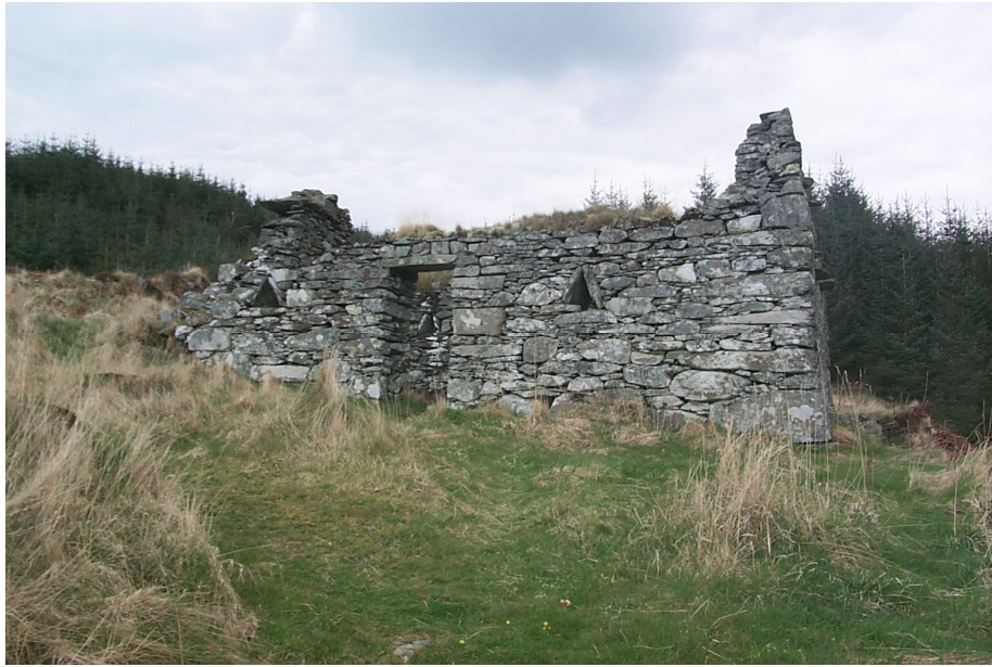
Figure 5.4 Barn with triangular vents and opposing doorways at Arichonan
