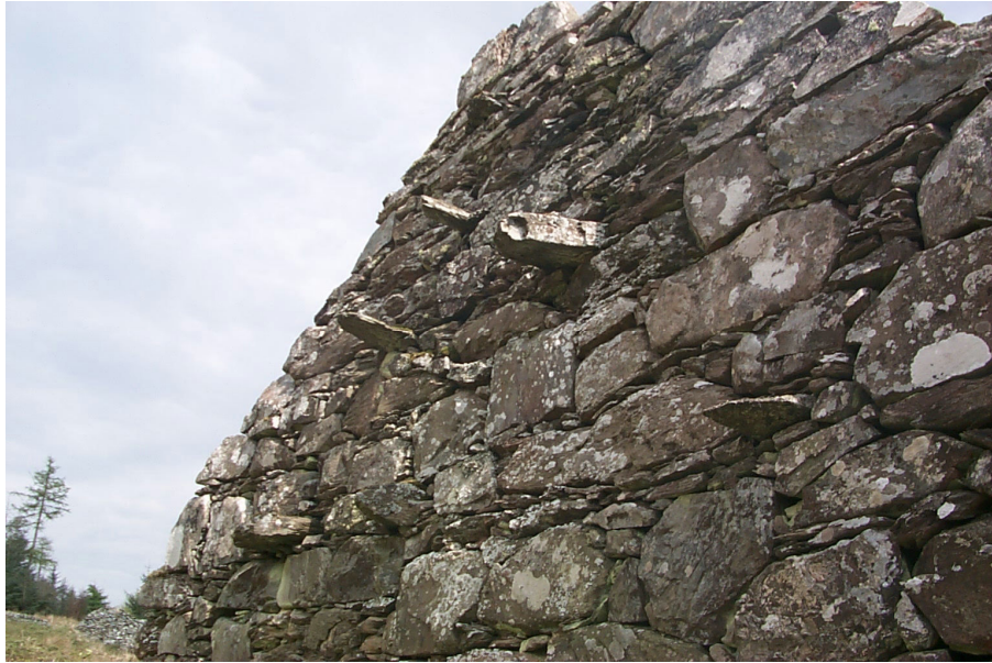
Figure 5.10 Arichonan Structure A1 gable with protruding stones for attaching the thatch
