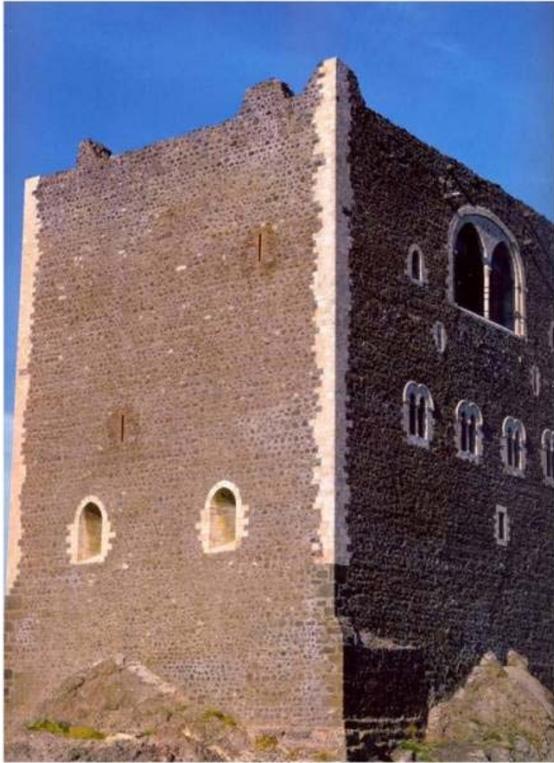
The donjon at Paterno, west of Catania, begun by Roger I in 1073. It is one of the few such structures that has remained unchanged throughout the centuries.
