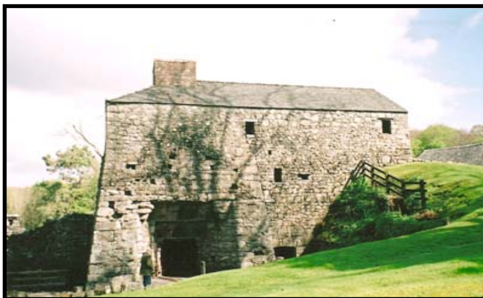
Cold-blast furnace used in the process of iron smelting at Bonawe, Argyll-shire from 1753 until 1876. At its height, the ironworks employed over 600 people, most of them Gaelic-speaking local inhabitants 'coaling' in the woods. Owned by a Cumbrian firm, the furnace itself was operated by skilled and semi-skilled English-speaking workers from the south. An example of a durable industry that benefitted crofters at nearby Taynuilt during the famine years of the mid-nineteenth-century. (Photo - JRS).
