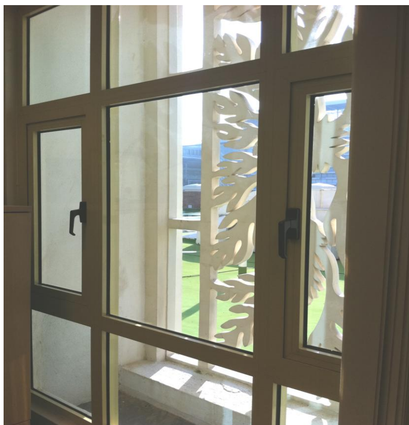
Figure 4-38: An example of a window in BHEUU, with its solar shading louver, taken at a time when the sun shone directly into it
