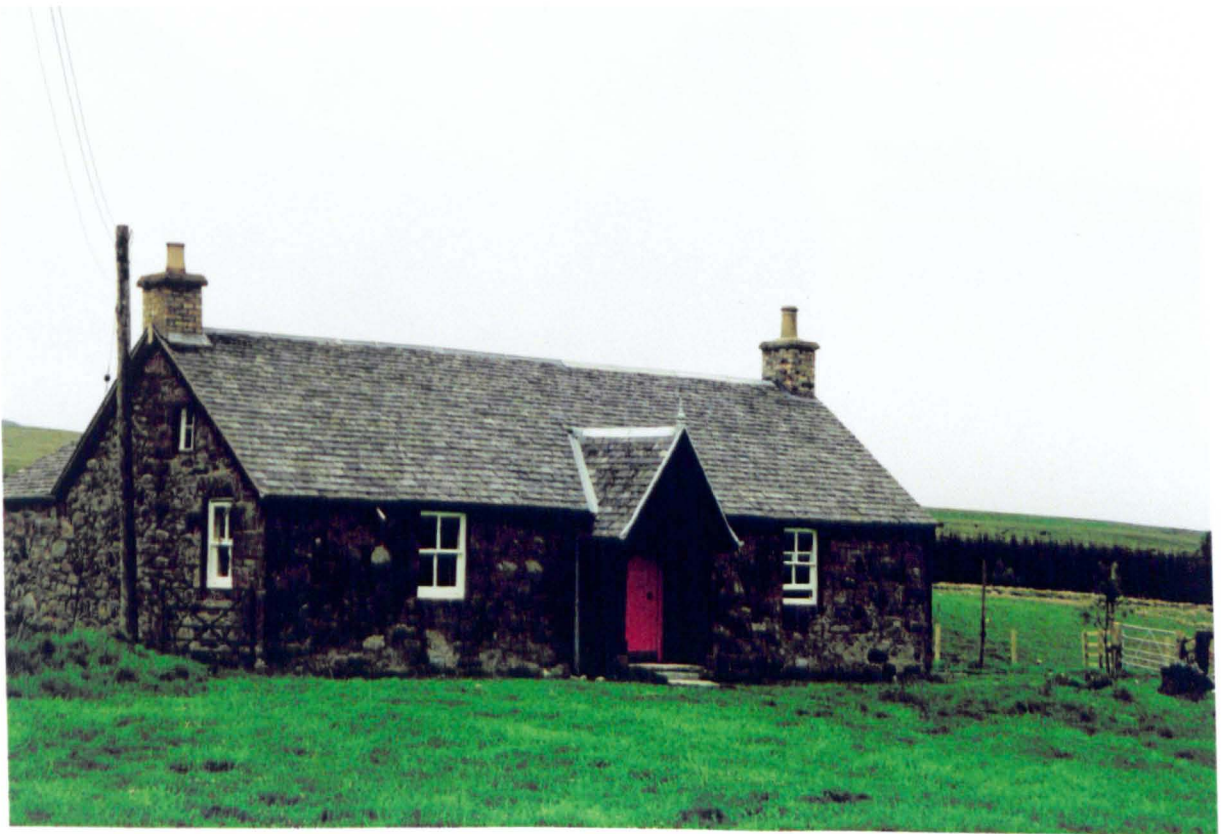
Plate 28 a & b Two adjacent buildings were roofed with slate from Craiglea Quarry, Logiealmond in the 19th century. a) The barn at Frances Field (Kipney) is now suffering from nail sickness. b) Bonellas Cottage has recently been reroofed using the original slate with less than 10% wastage.
