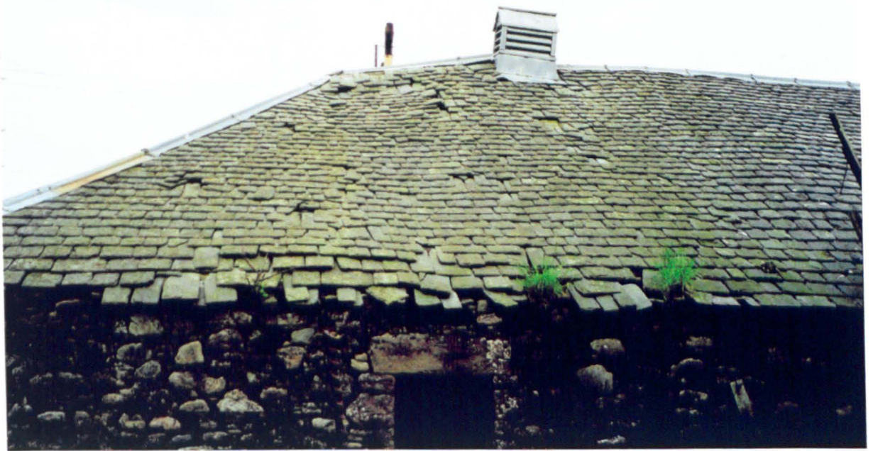
Plate 28 a & b Two adjacent buildings were roofed with slate from Craiglea Quarry, Logiealmond in the 19th century. a) The barn at Frances Field (Kipney) is now suffering from nail sickness. b) Bonellas Cottage has recently been reroofed using the original slate with less than 10% wastage.
