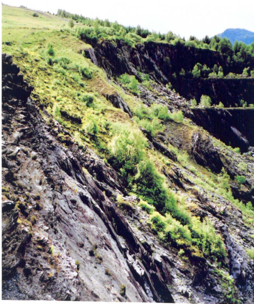
Plate 3 East Laroach -View of the landslide on the SE of the quarry
