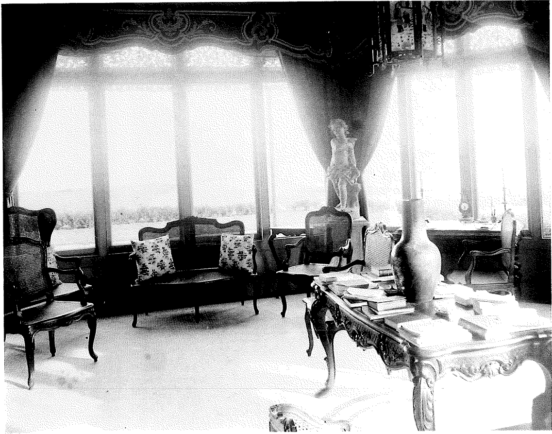
Plate 66. Glass Room, Land's End, c.1900
