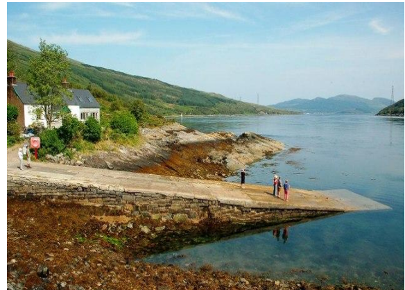
Figure 33: Pier at Kylerhea
