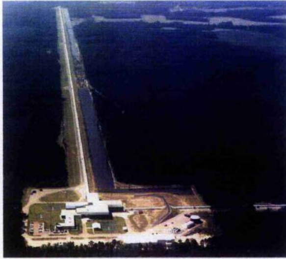
Figure 1.4: One of the LIGO gravitational wave detectors in Livingston, Louisiana. The other detector is over 3000km away in Richland, Washington. The arms of both detector are four km long and are housed in an ultrahigh vacuum system. Using two detectors the detection of a signal can be validated, and the origin can be determined.
