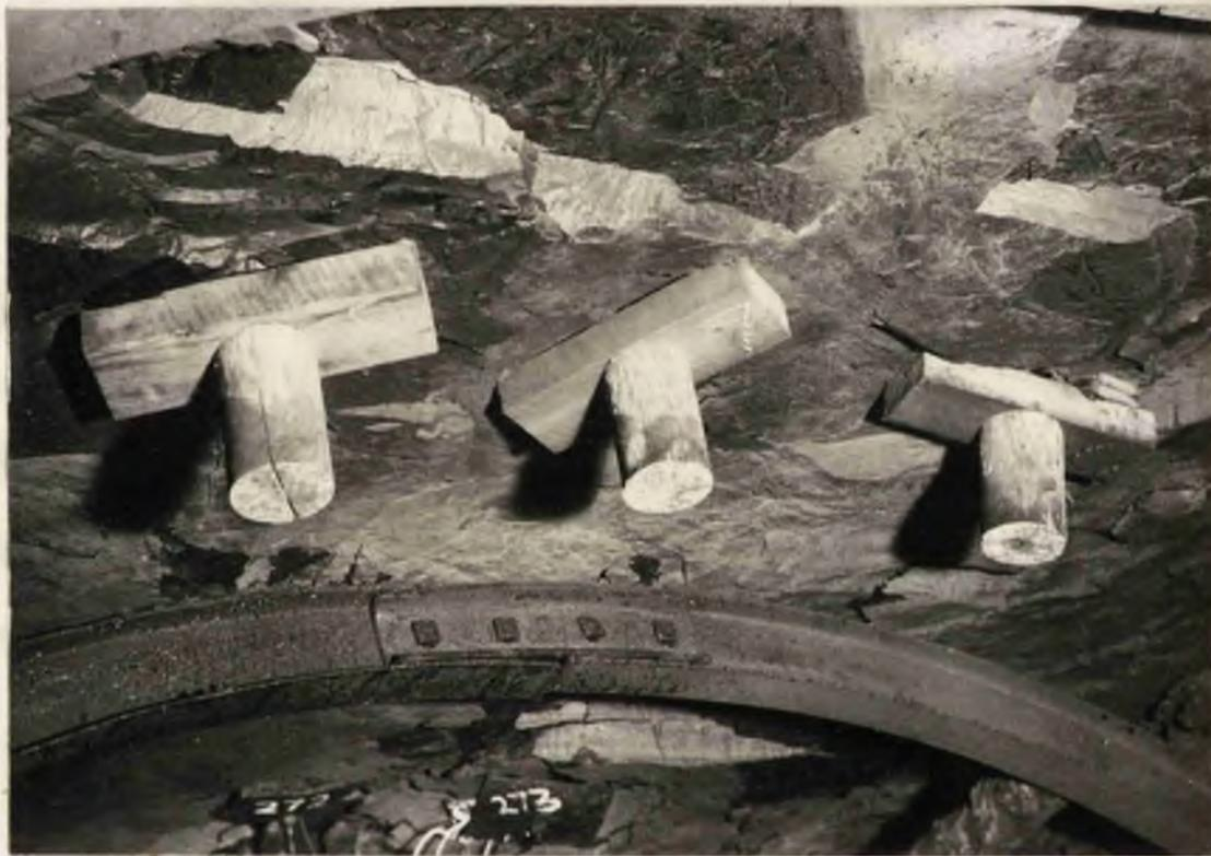
14th May. 1955. There is no marked breaking-up of the roof between the bolts. The wedges between the plates and the roof show sign of weighting.
