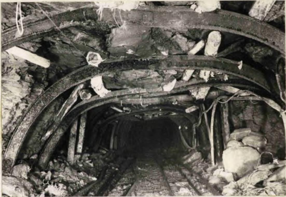
16th March, 1955. This plate shows the conditions in the unbolted roadway. The failure of the immediate roof bed is clearly seen; resulting in large amounts of fallen debris which has to be cleared to the roadsides. Part of the roadway which has been re-ripped can be seen in the background.
