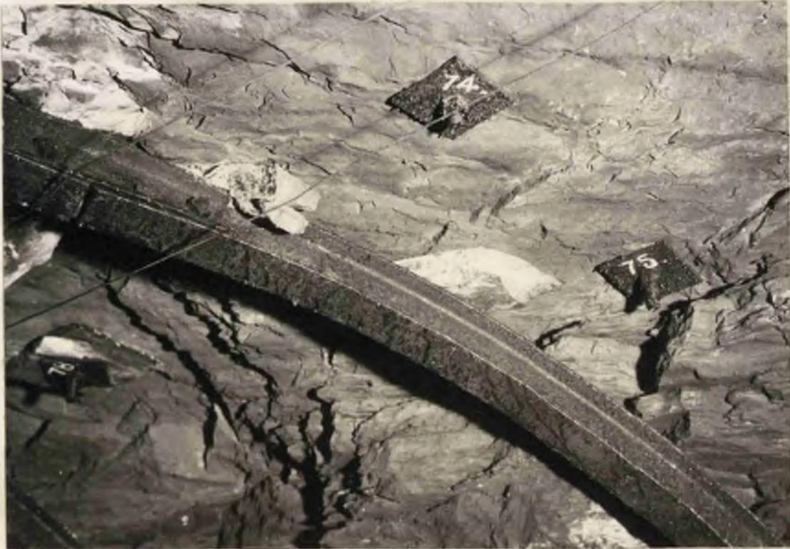
14th May, 1954. The immediate roof bed shows no sign of failure and there is no distortion of the girders after five months. The roof has lowered, as the wood block between the girder and the roof is severely crushed.
