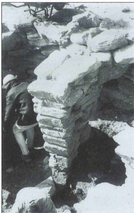
Plate 25: Remains of a pier at Cnip built from gradually wider stone blocks (from Armit 2003, 139).
