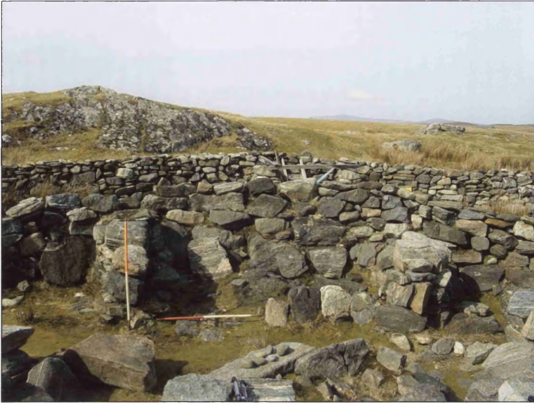
Plate 33: View from central wheelhouse space of bay two with piers H (left) and G (right) some 3.6metres apart.
