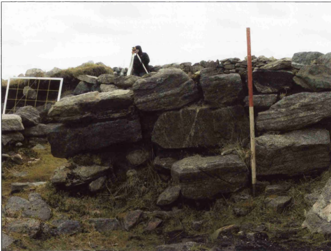
Plate 34: Pier H viewed from within bay two showing protruding 'bench' stones.
