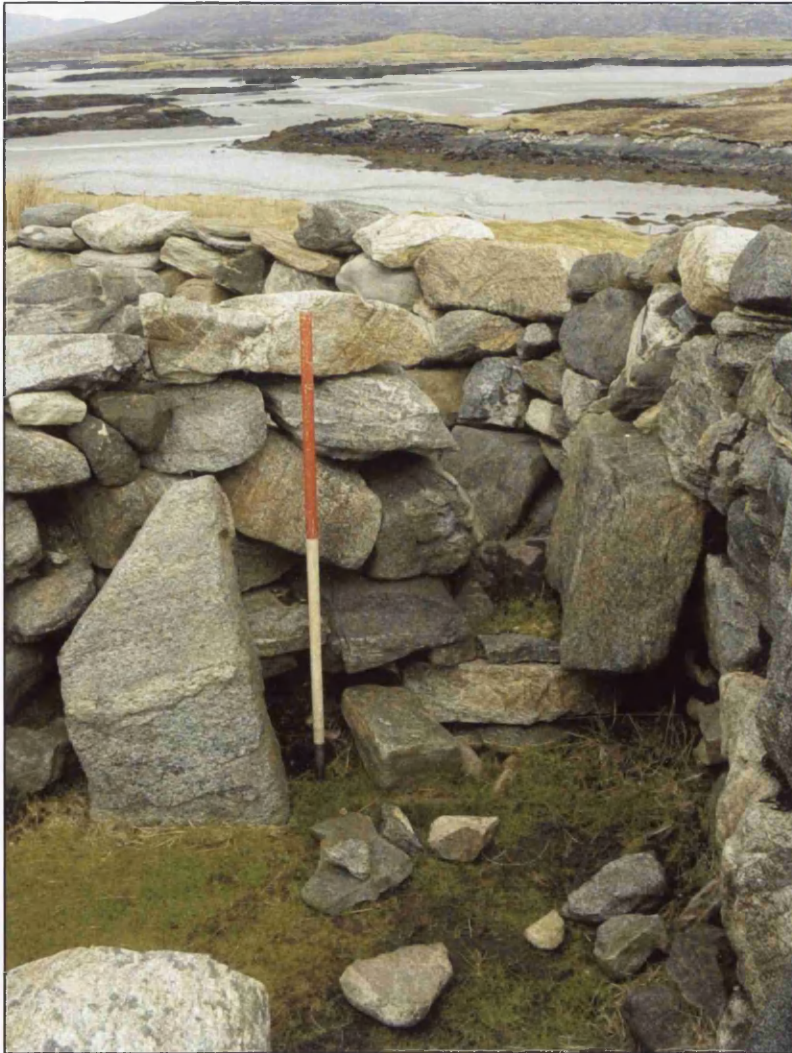
Plate 23: View from bay six of the aisle behind pier D with bonded and protruding stonework.
