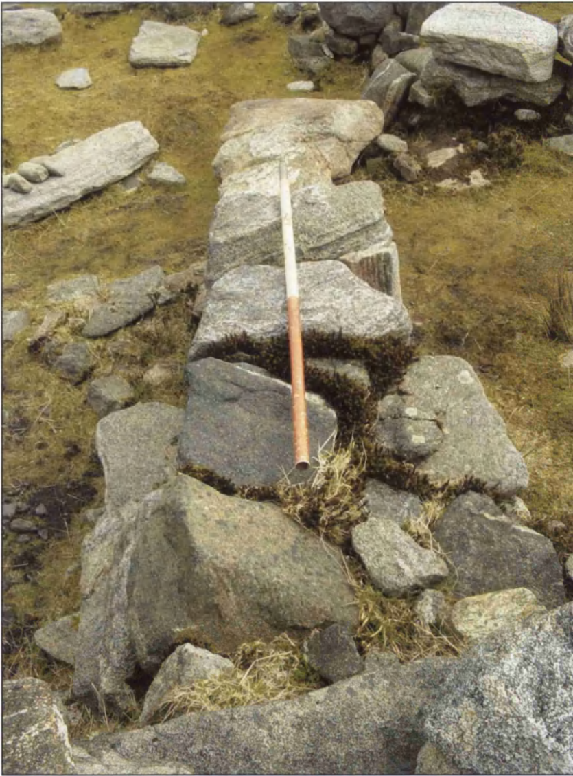
Plate 32: View of pier H from the outer wheelhouse wall where it meets the pier inner face.
