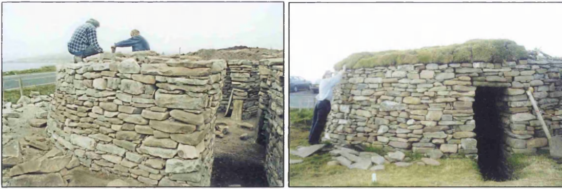
Plate 46: Experimental construction of a freestanding wheelhouse at Scatness, Orkney.
