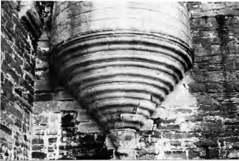
Plate 11 : Kirkwall, Earl's Palace, circular corbelling.
