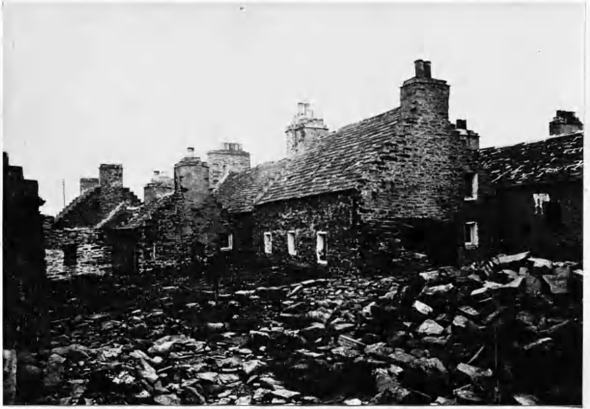
Plate 73 : Kirkwall, Shore Street lane, 20th century.
