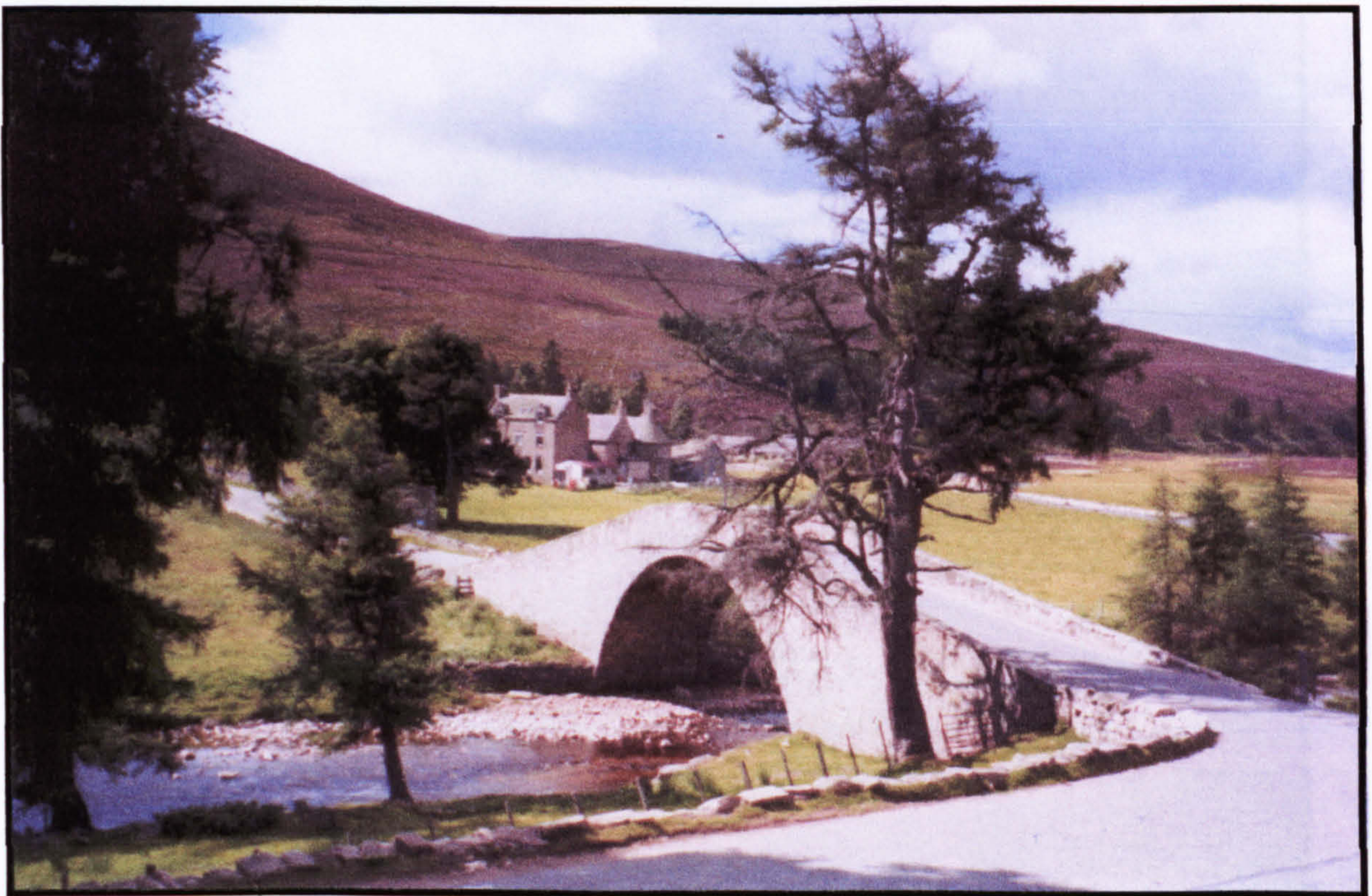
Gairnshiel Bridge, (Caulfeild era), upper Deeside, Aberdeen-shire. The bridge's solid construction has withstood two-and-a-half centuries of heavy wheeled traffic. (photo-JRS).
