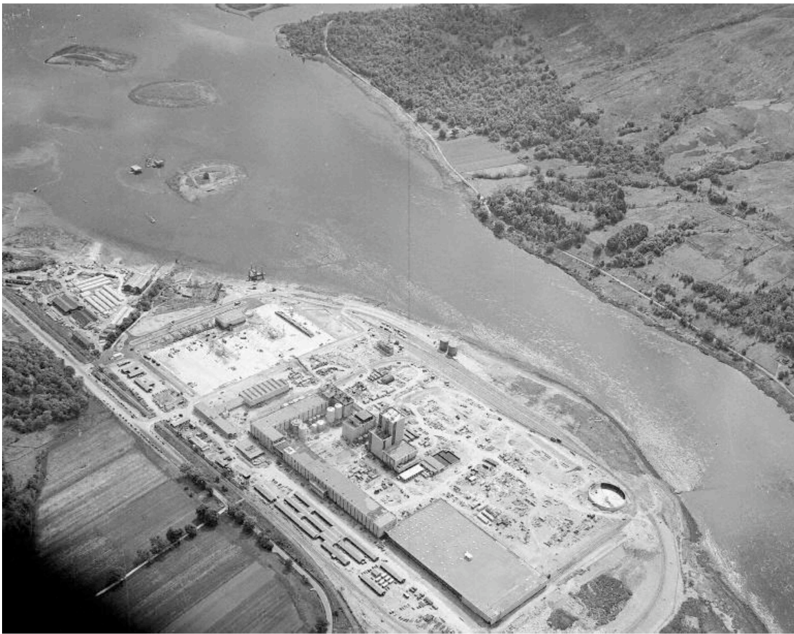
Figure 2.2 Construction phase of the Corpach mill development
