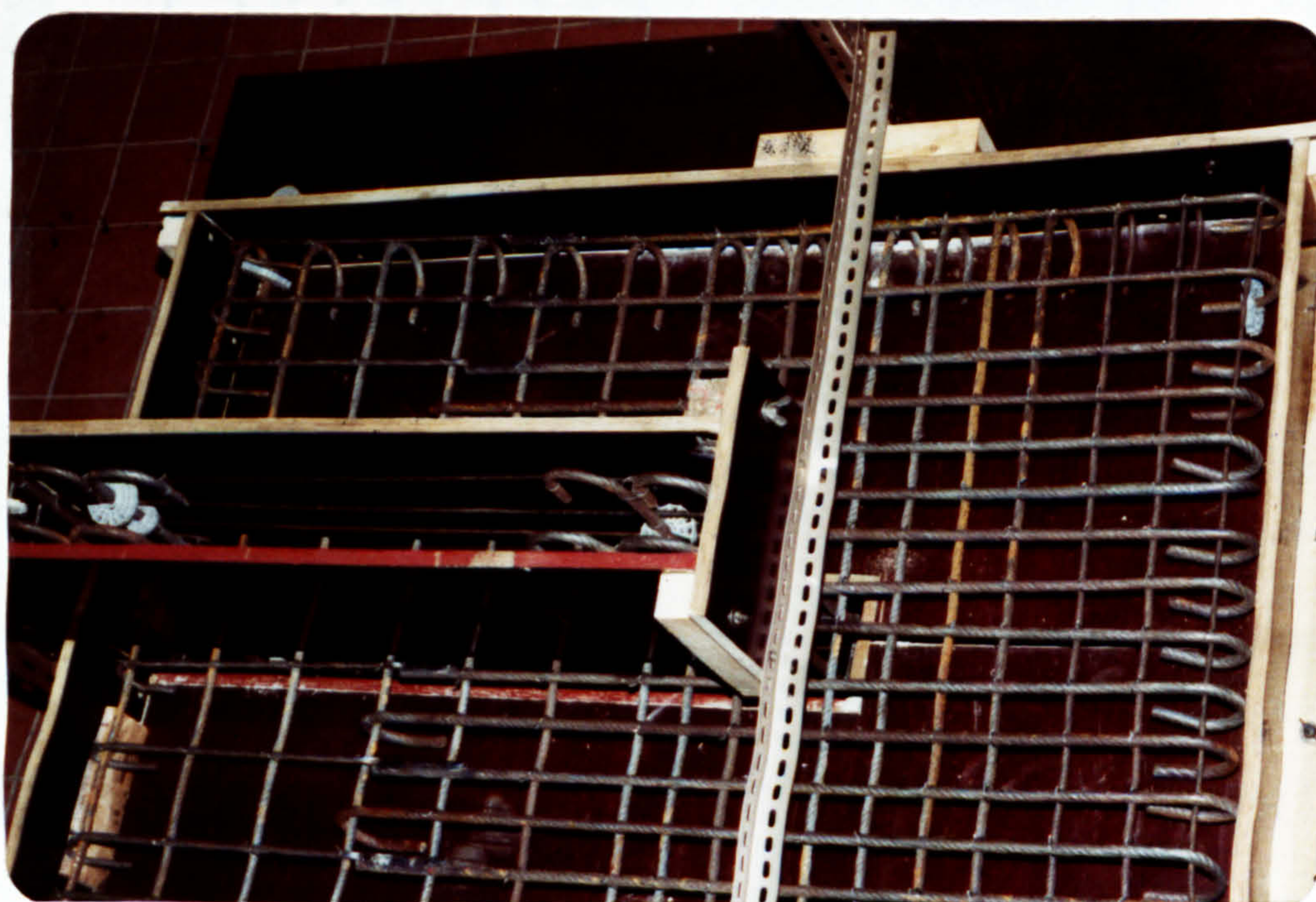
Figure (6.41) : Photograph showing the arrangement of steel in model MT1 .
