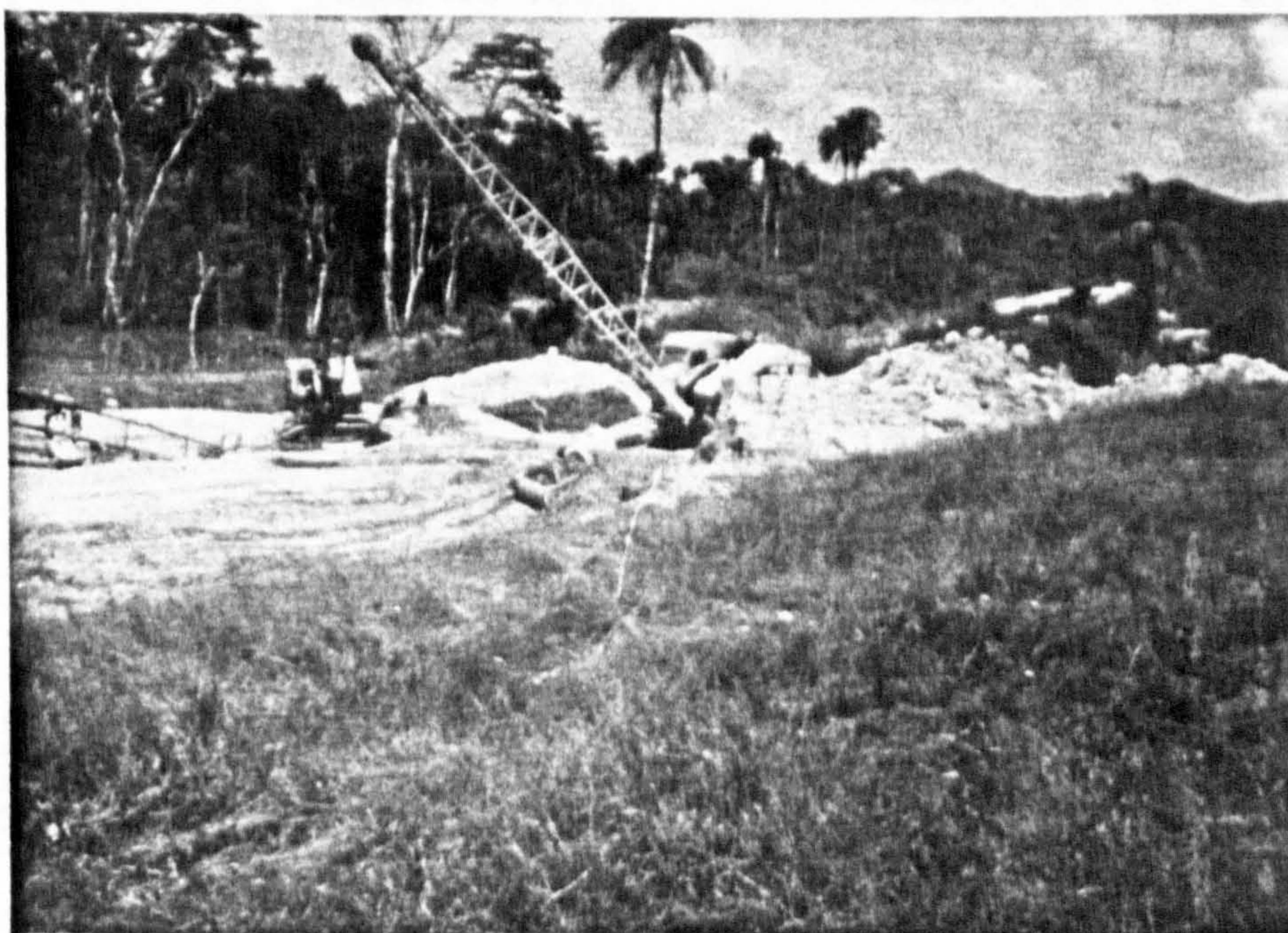
Illustration 12: A dragline (RB 22) in operation, seen here loading diamondiferous gravel on to the conveyor-belt supplying S.L.S.T.'s No. 9 Plant: Tongo Field, Kenema District (November 1968).
