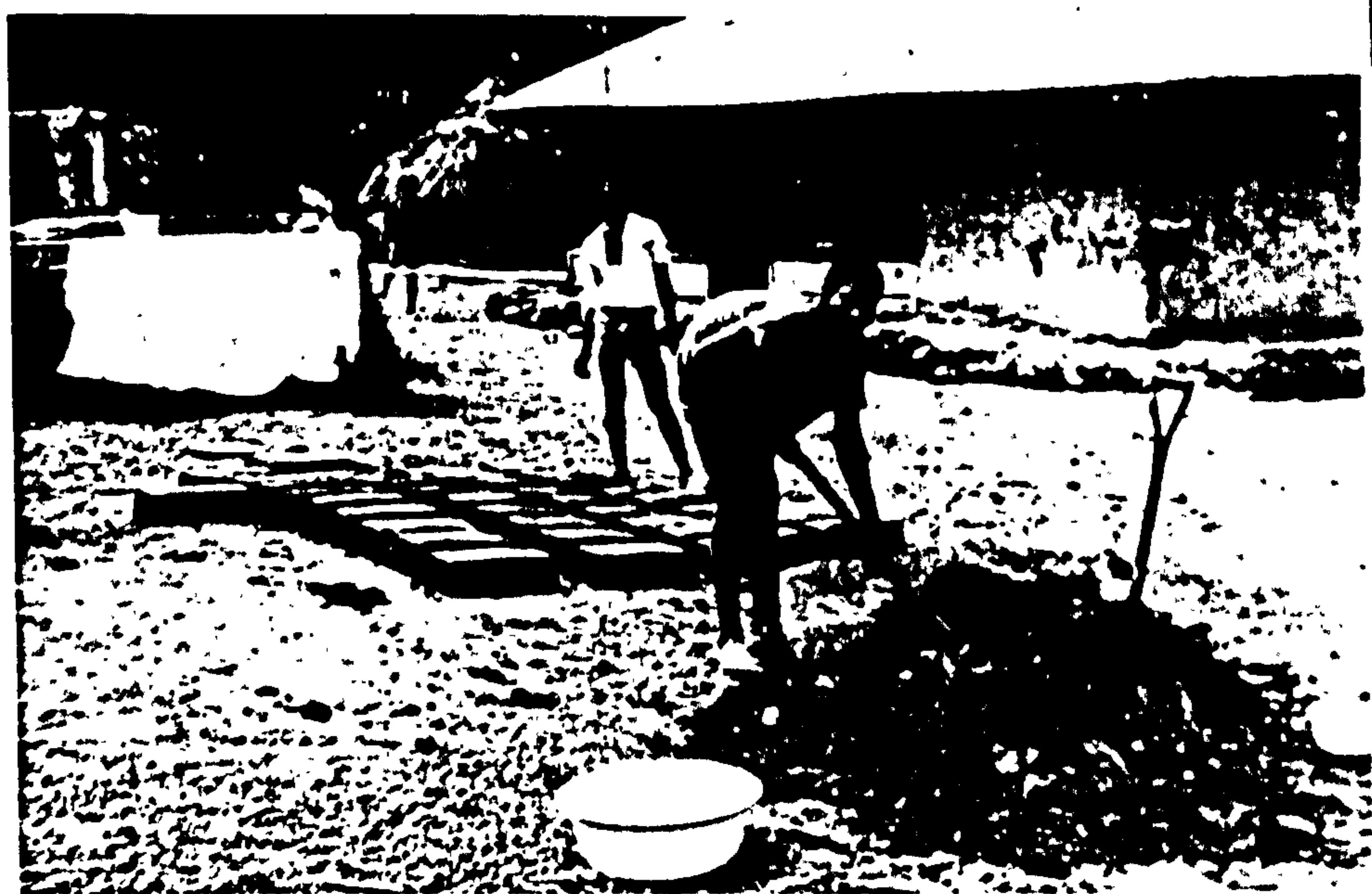
Illustration 2: Mud-block making for house construction: Dandaya Village, Sambaia Chiefdom, Tonkolili District (March 1973).
