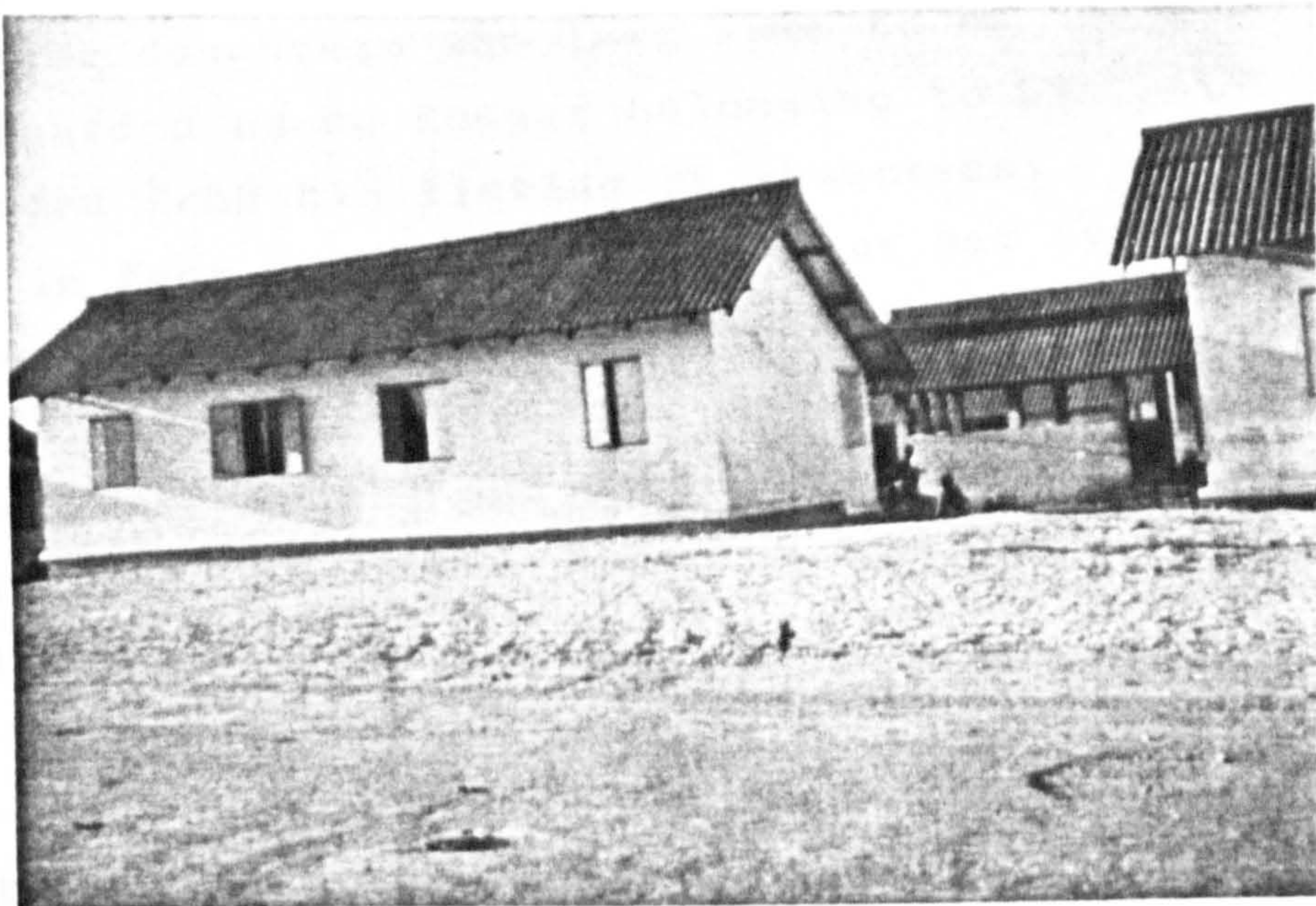
Illustration 25: S.L.S.T. company lines; a concrete walled and corrugated-iron roofed four unit block: Koidu Town, Kono District (October 1968).
