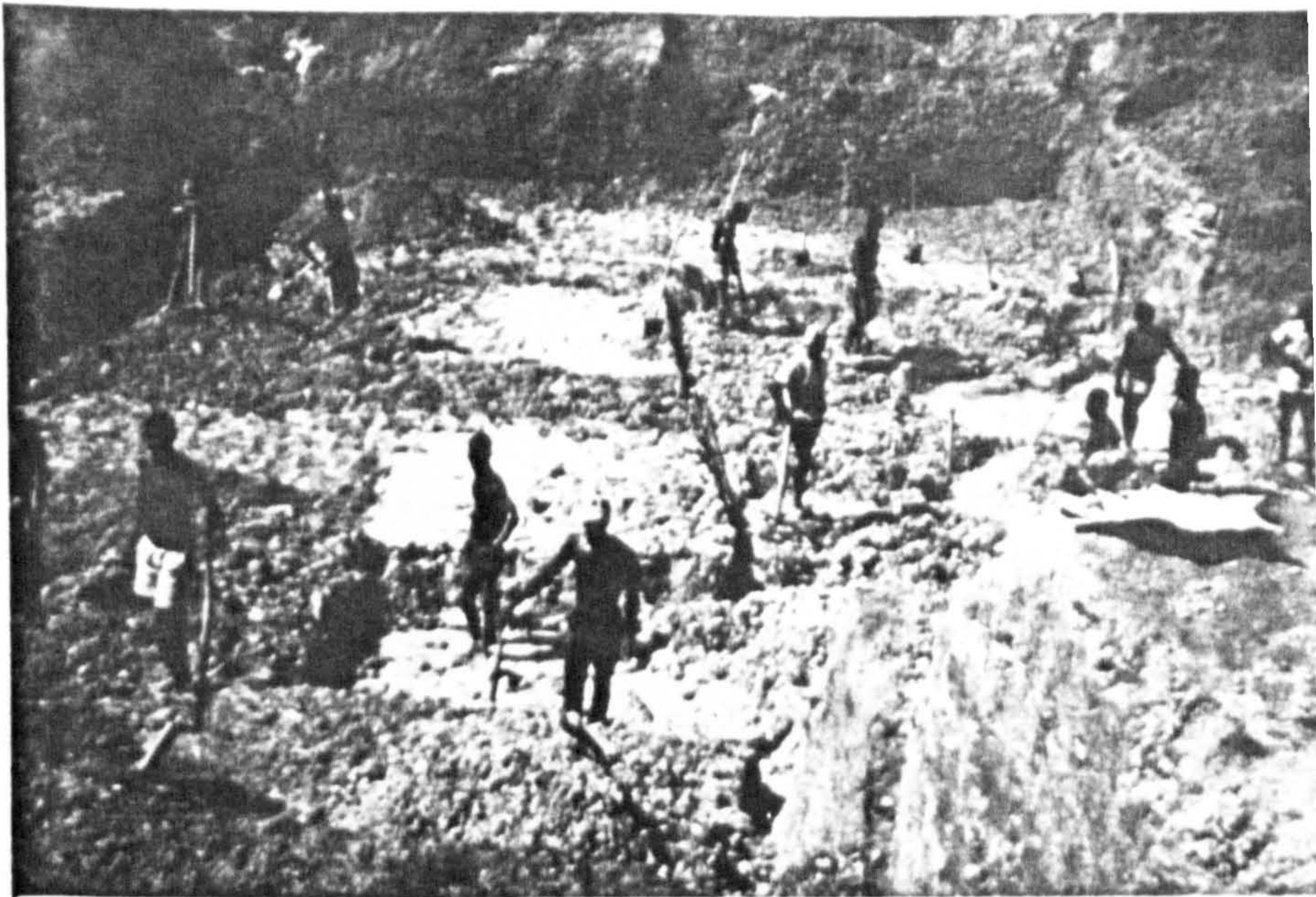
Illustration 15: A well-ordered licensed mining plot indicates how close supervision by mines wardens can produce safe working conditions even when considerable overburden has to be removed: Yomandu, Sando Chiefdom, Kono District (January 1969).
