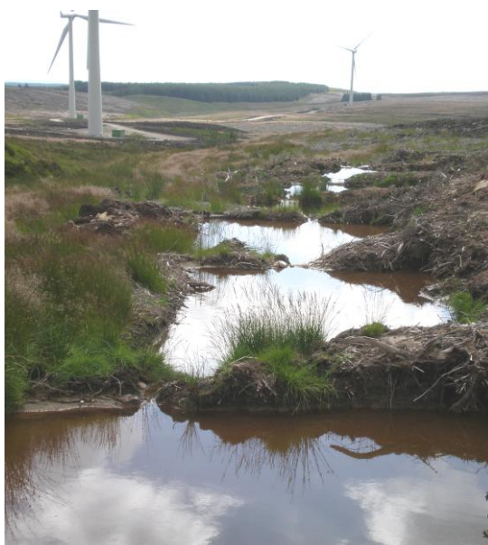
Figure 36. Use of settling ponds at Whitelee to increase the retention time of the water in the catchment so that the suspended load settles out as a mitigation measure to prevent suspended solids and consequently POC reaching streamwater.
