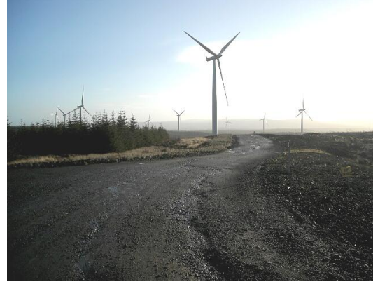
Figure A2. Floating road design access track with cable trenches parallel to road lines.
