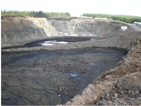
Figure A1. Borrow pit (onsite quarry) where stone has been removed and then backfilled with peat.
