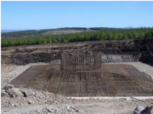
Figure A3. Excavation for installation of turbine foundation. Photo courtesy of Scottish Power.
