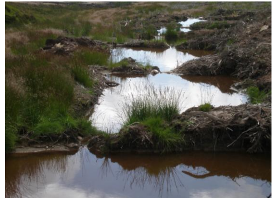
Figure A4. Sediment settling ponds as a water quality mitigation measure.
