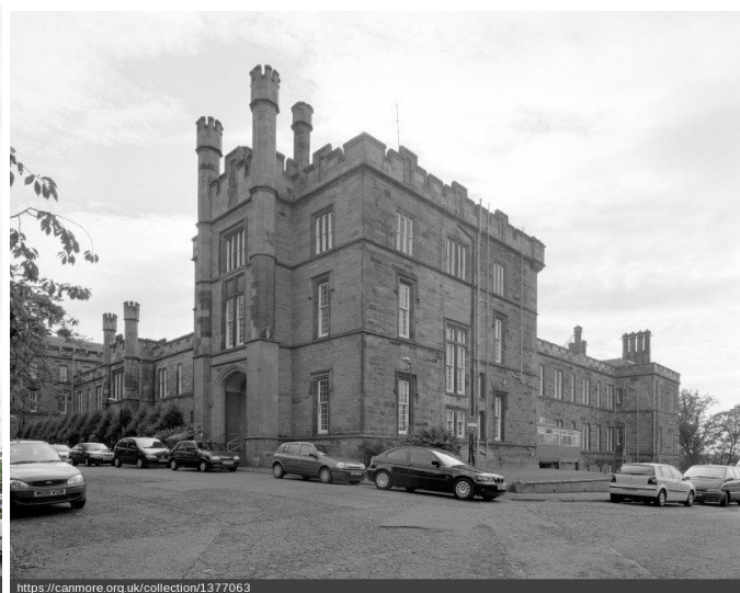
Figure (3.9), Gartnavel hospital building. (Canmore)
