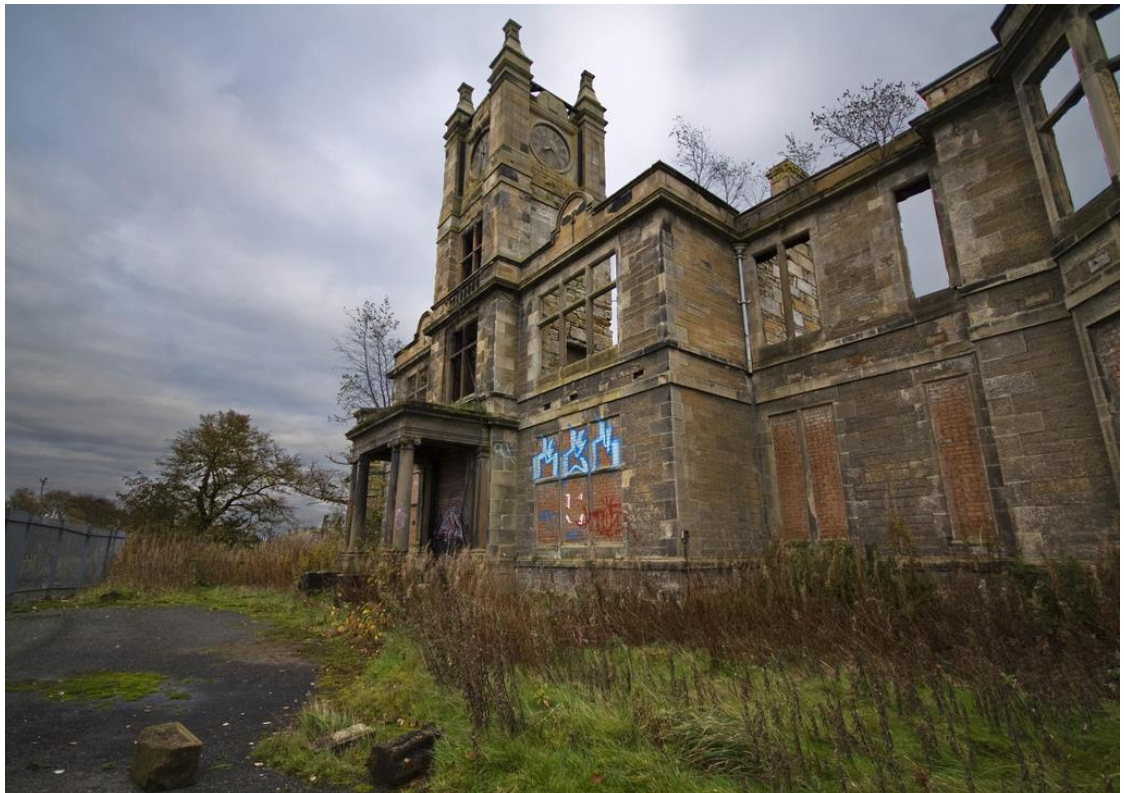
Figure (5.6). Ruins of Woodilee prior to renovation, with vandalised and graffitied exterior (MacPherson, 2009)
