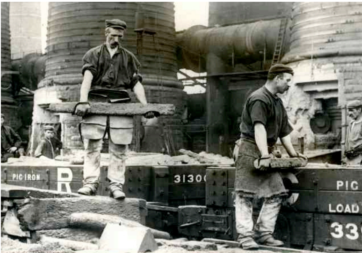
Figure 4 - Breaking pig bars. Coltness Iron Works in 1900 - 1910. Photograph courtesy of Motherwell Heritage Centre.
