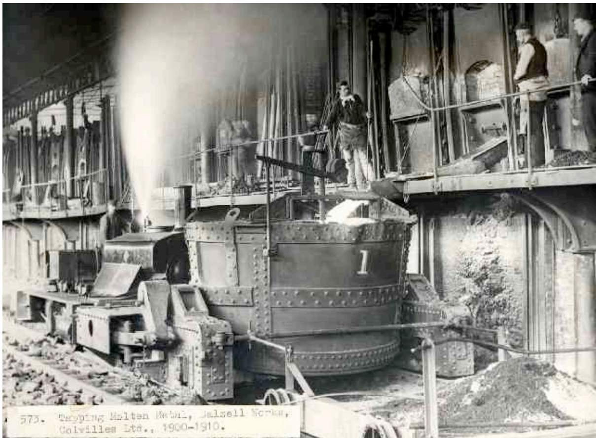
Figure 6 – Tapping Molten Metal, Dalzell Works, Colvilles Ltd., 1900 – 1910. Photograph Courtesy of Motherwell Heritage Centre.
