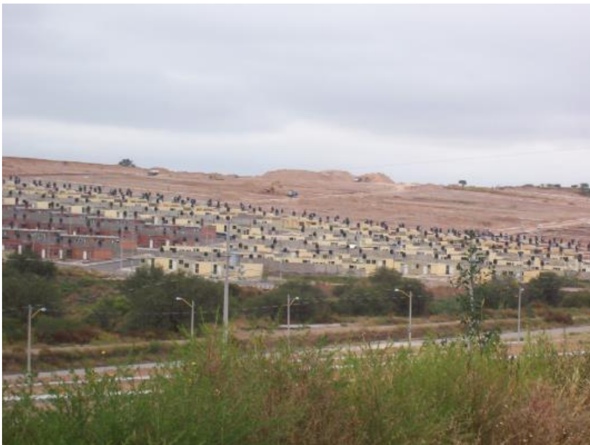
Figure No. 96. A view of a formal housing area under construction.
