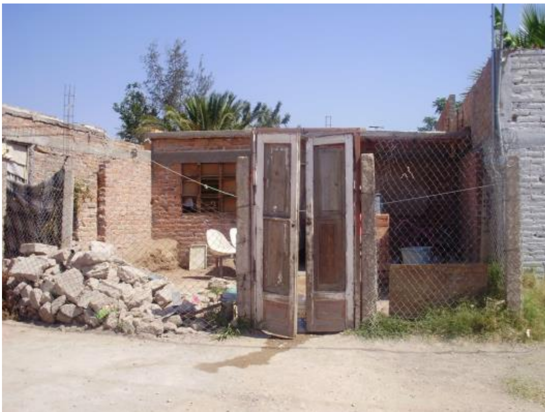
Figure No. 70. LP-06 protected as much as possible from intruders.
