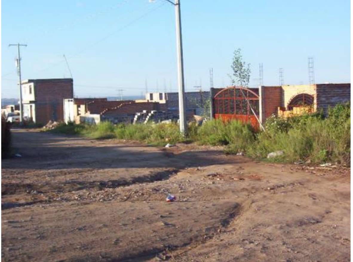
Figure No. 83. Electricity posts along unpaved streets in Paso Hondo.
