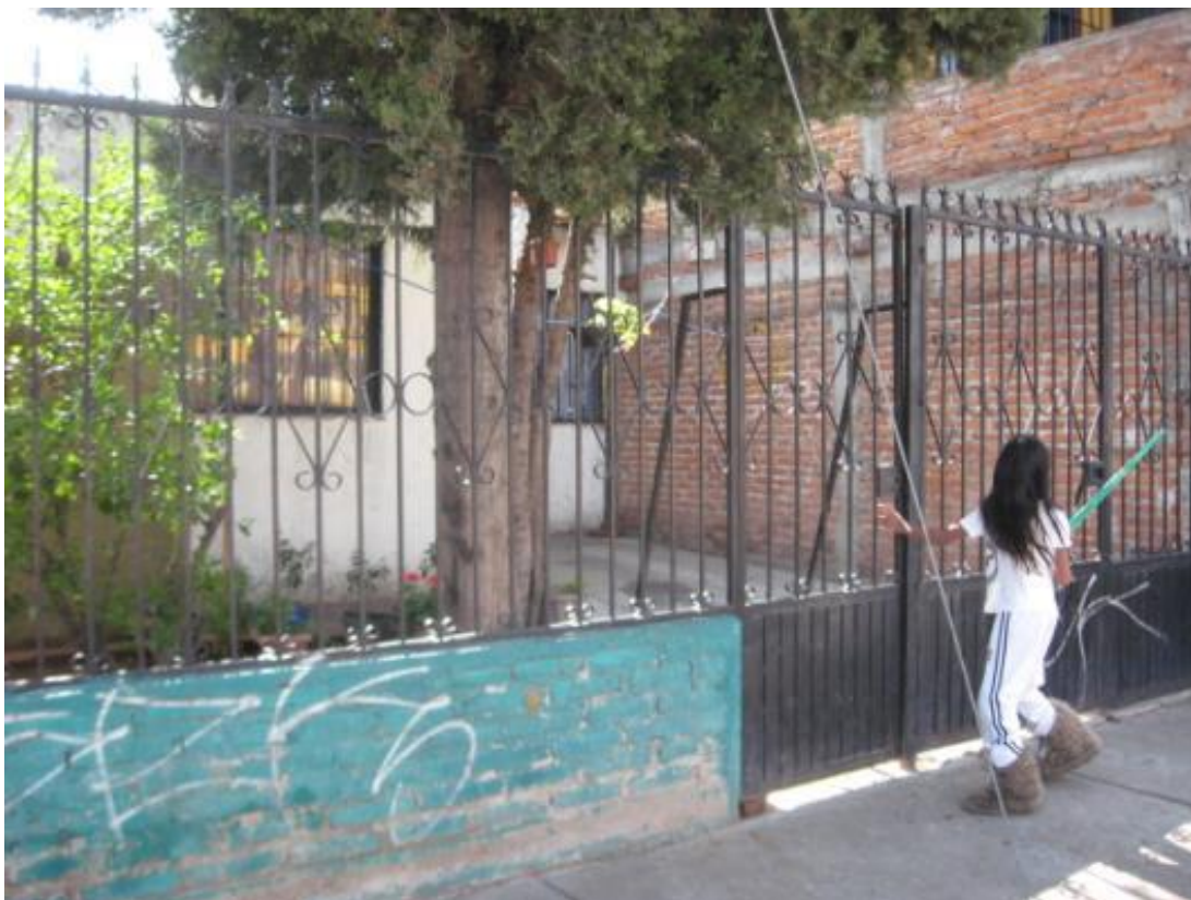
Figure No. 71. The MO-01 façade protected by steel bars/spikes on top.
