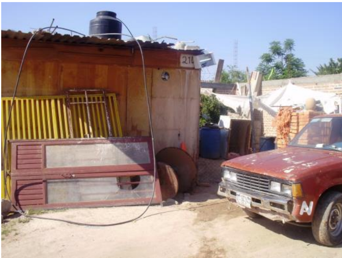
Figure No. 21. A house in the process of consolidation process. Source: Carlos Hernandez–Velasco (2010).
