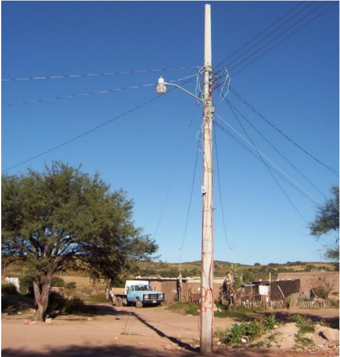
Figure No. 81. Illegal electricity connections to a lamppost in Paso Hondo. Source: Carlos Hernandez–Velasco (2009).
