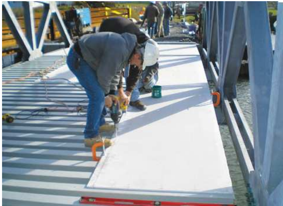
Figure 2.8: Pultruded composite bridge [30]
