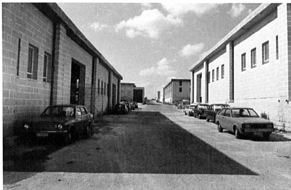
PLATE 9.1 Bulebel Industrial Estate. This is the largest of the Government industrial estates. The factories are constructed from the uniform globigerina limestone blocks quarried locally (see plates 5.3 and 5.4), and the steel substructures are usually manufactured in the dockyards of the Grand Harbour.
