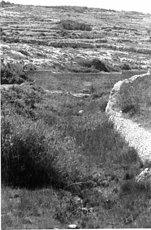
PLATE 5.1 A Dam Located in a Maltese Wied (dry valley). This is one of many dams designed to arrest storm runoff which would otherwise flow away straight into the Mediterranean. By reducing such runoff, dams such as this allow rainwater to infiltrate downwards through the geological strata, recharging the aquifers.
