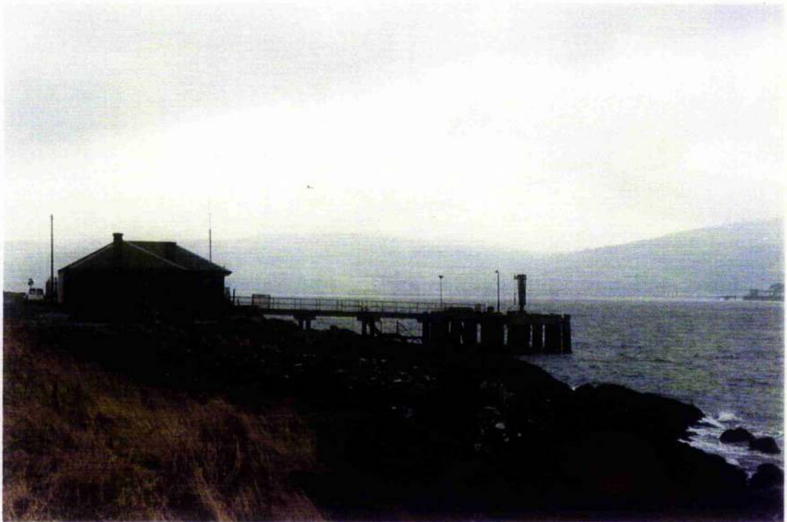
Fig. 4.2.4 Keppel Pier, January 1996.
