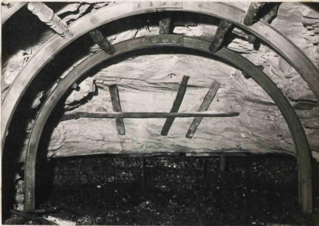
Ripping Lip (supports removed) showing marked change in strata conditions. Note the current bedding in the massive sandstone.
