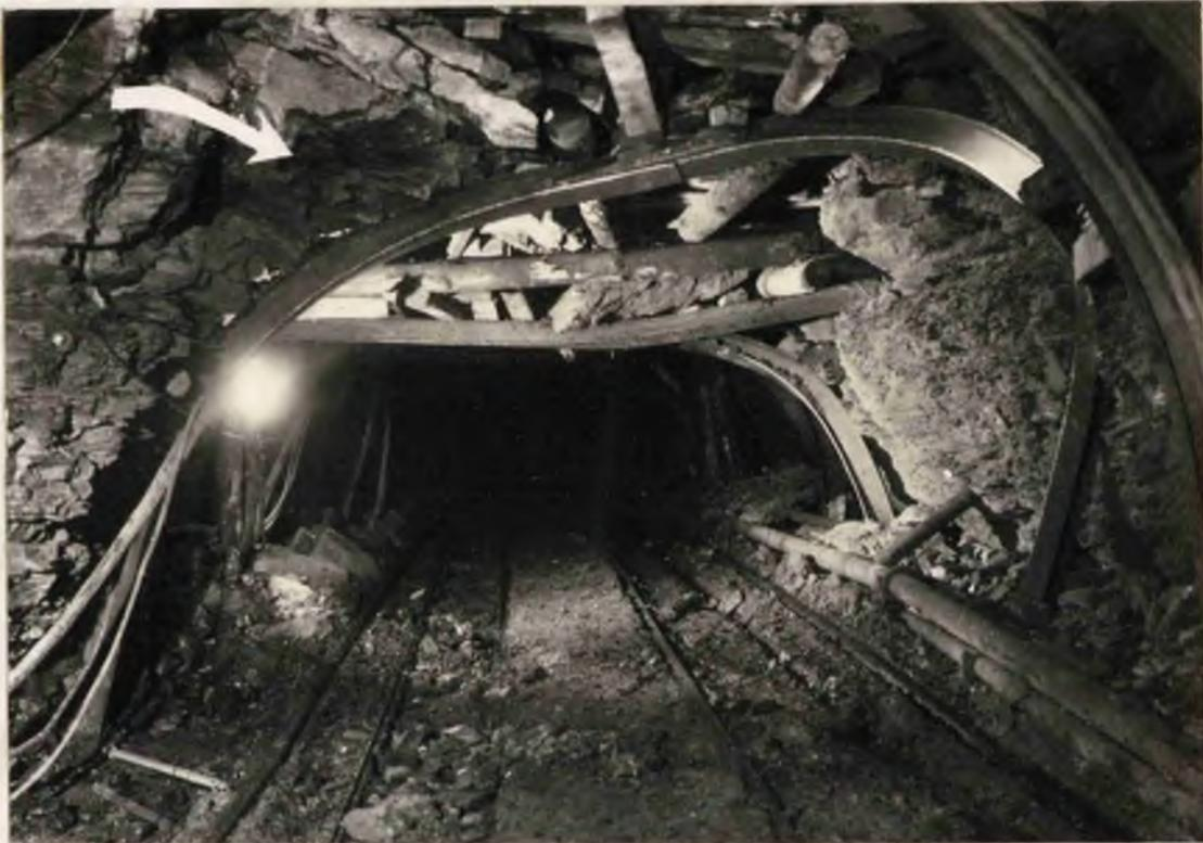
16th March. 1955. Looking inbye from the re-ripped length towards the unbolted roadway. The excessive roof lowering is clearly seen and also the complete failure of immediate roof over the centre of the excavation - resulting in movement of the sides into the roadway. (Compare this plate with the results obtained in the laboratory plaster model tests later.)
