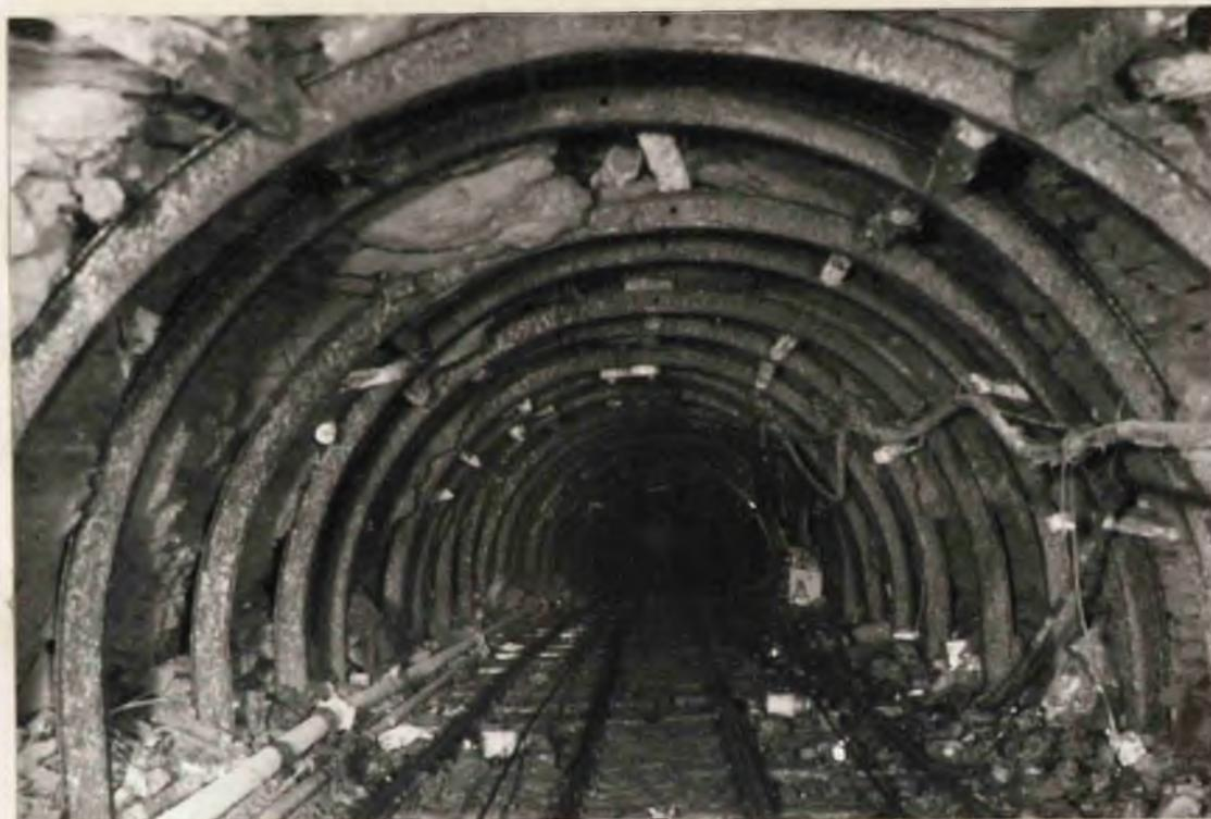
14th May, 1955. Looking outbye towards the wedge-bolted section. The girders are not distorted to any extent, and the immediate roof bed has remained intact. Note particularly the absence of fallen rock at the roadsides and the small amount of timber used with the girders.
