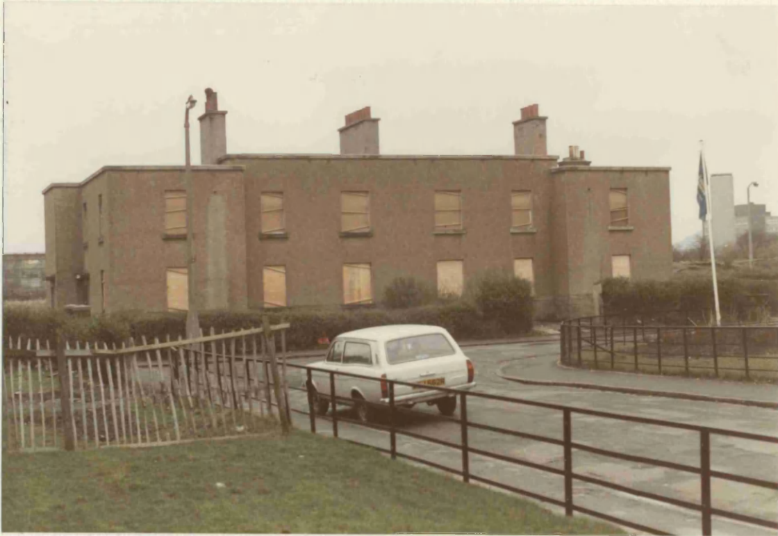
WEST PILTON, EDINBURGH. Unmodernised block.
