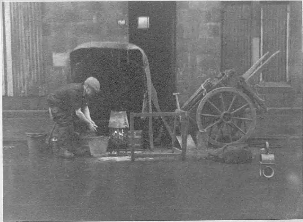
Fig. 1. : Working Site [Surface].
