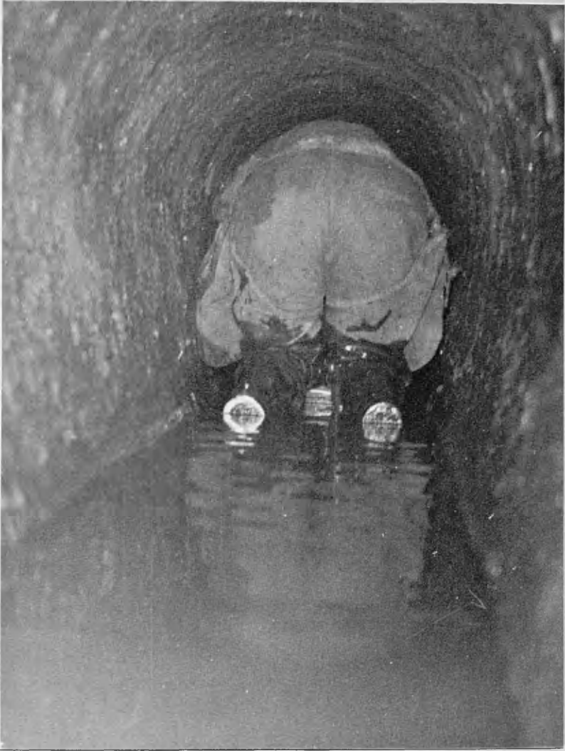
Fig. 5 : Fitting Bucket [Back View] (3'-6" Sewer).
