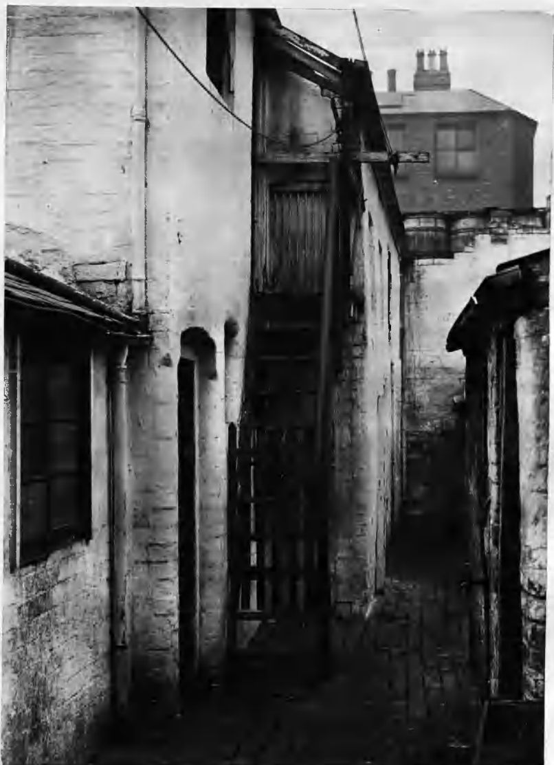
13. The cleanest premises inspected (No 6 in Table 2).
