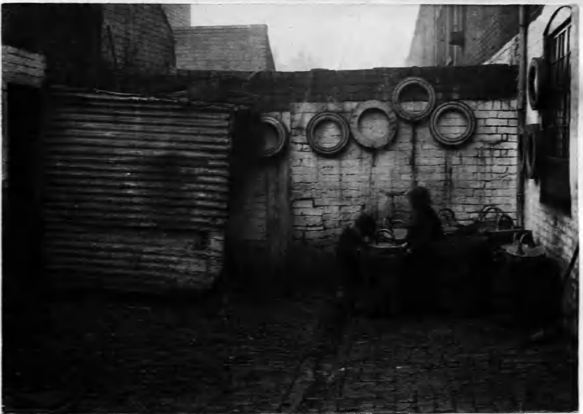
7. Interior of shed shewn in Photograph 6.
