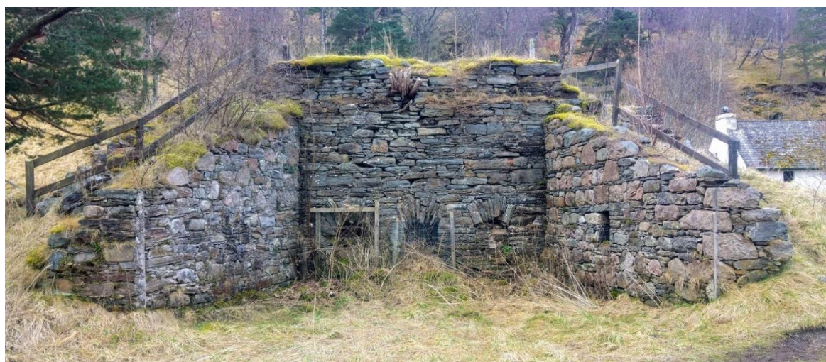
Figure 54 Draw kiln at Loch an Eilein, Rothiemurchus. A small limestone quarry is located a short distance up the hill behind the kiln. Note the long buttresses on either side, which likely offered support for the kiln facing.
