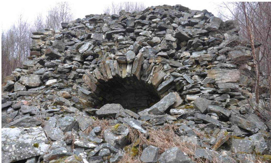
Figure 52 Lime kiln in Rothiemurchus, indicating the difficulty of determining whether kilns were continuous or not from their remains. The kiln walls are of dry-stone construction, with the draw arch mortared. Photo: David Taylor.
