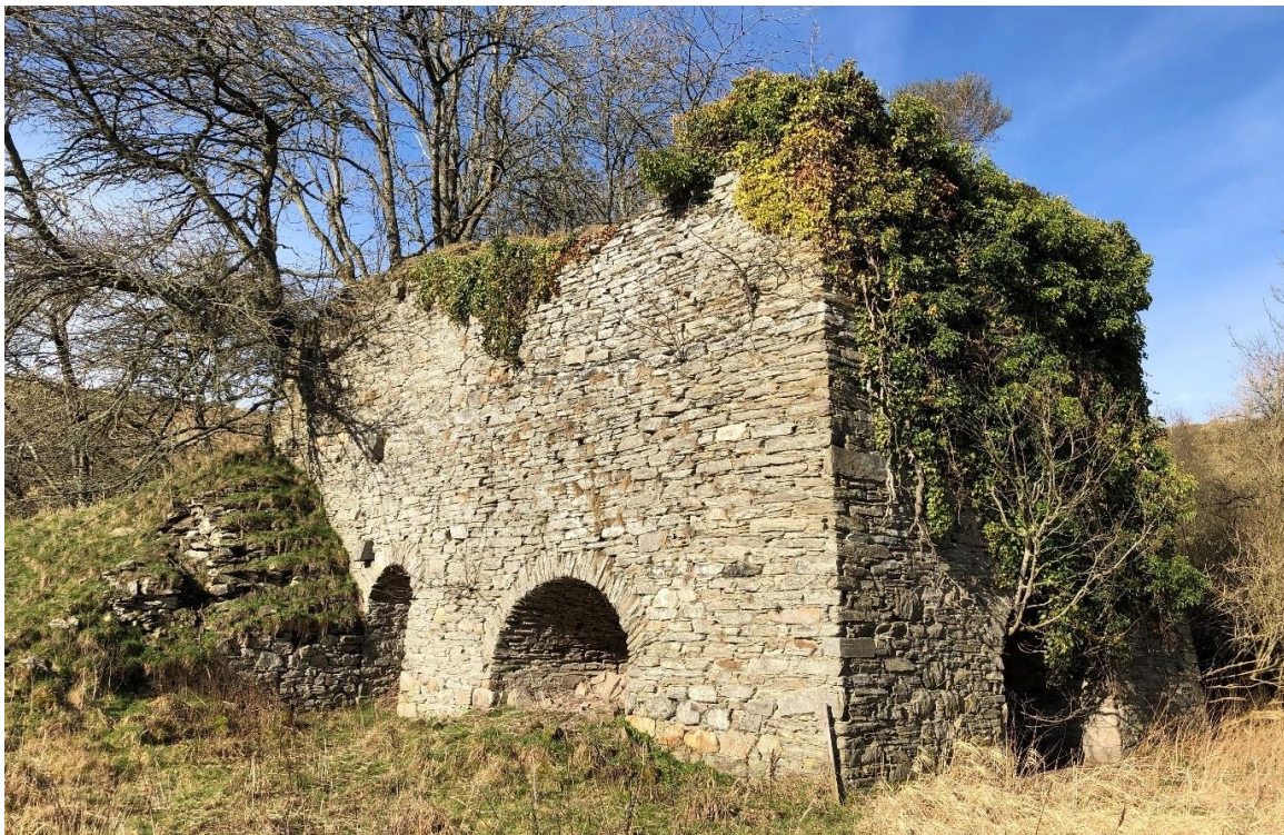
Figure 55 Northernmost and newest lime kiln at Ardonald lime works, measuring approximately 9m tall. Three draw holes are visible on each side of the kiln. A tunnel (now infilled) runs behind the pot and may have given access to a fourth draw hole. An adjoining building on the north side (not shown) was likely
