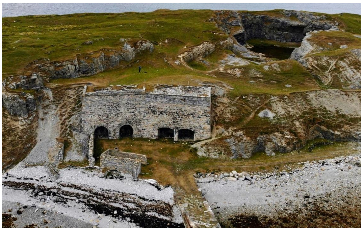
Figure 56 Bank of four draw kilns at Ard Neakie, Loch Eriboll, with pier in foreground and quarry to the rear. The different shape of the arches on the left and right of the kiln suggest that one side was built after the other, perhaps by different masons. Photo: Angus Mitchell.
