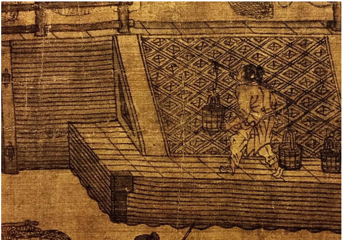
Figure 242 Detail of The Water Mill , the stairs with xiangyan
