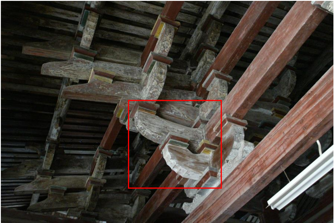
Figure 217 The double bracket-arms, Song The Sanqing Hall of the Yuanmiao Temple, Putian, Fujian province
