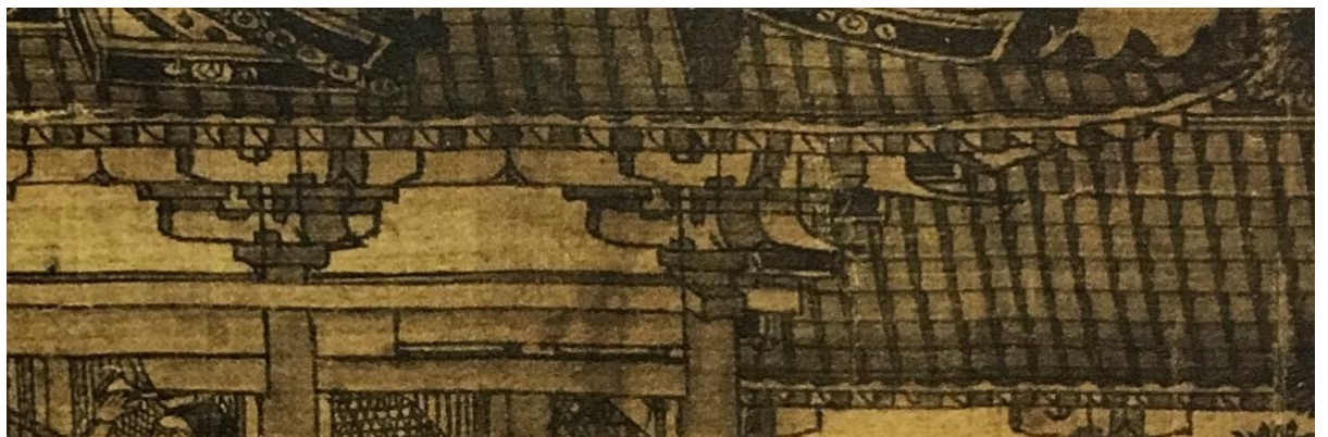
Figure 235 Detail of The Water Mill , the ang and shuatou of the water mill hall
