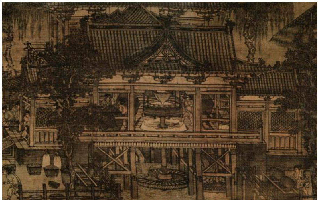
Figure 211 Detail of The Water Mill , the single-eave crossed hip-and-gable roof of the water mill hall
