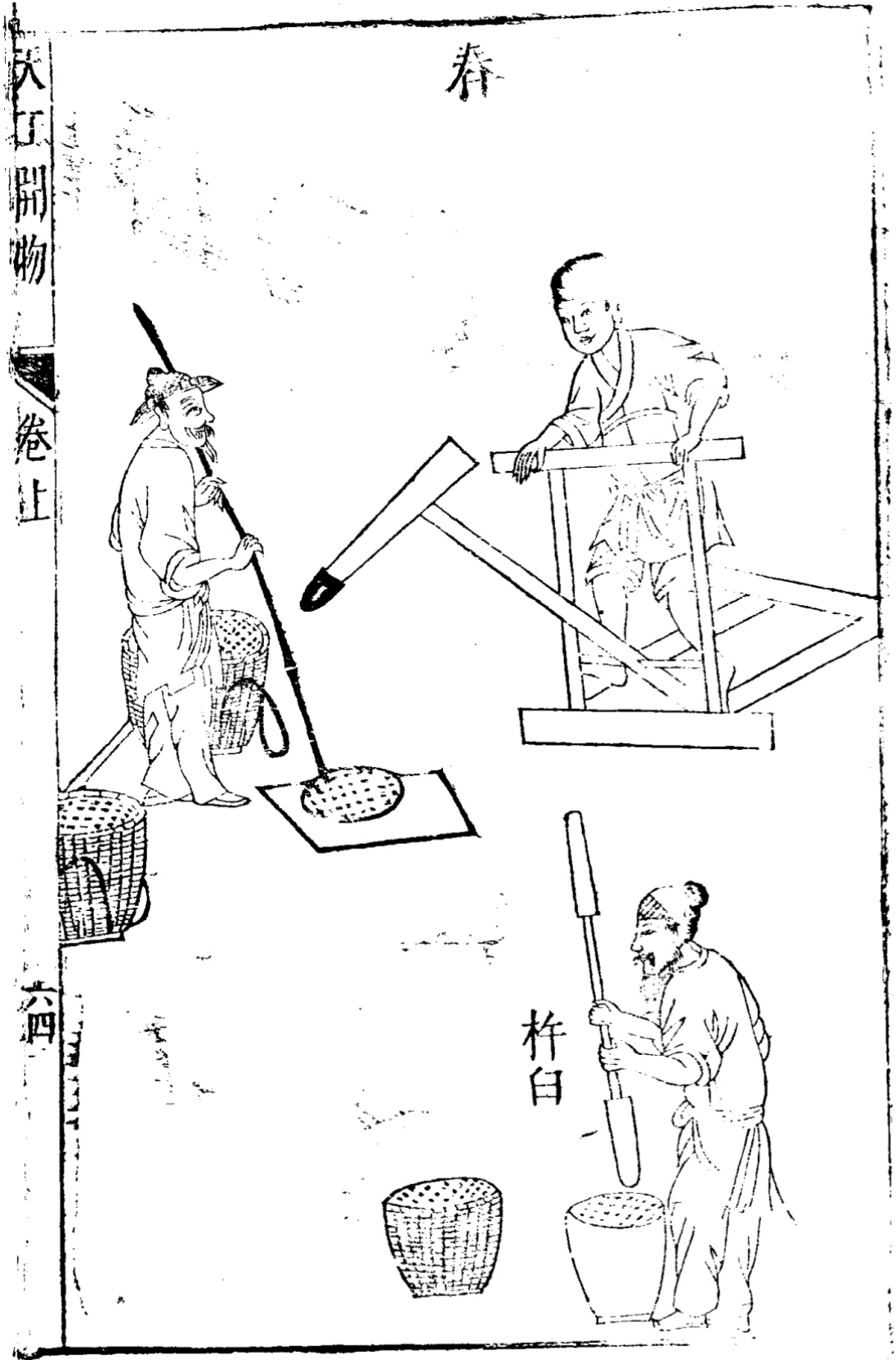
Figure 246 The chong (Image from Tiangong kaiwu , 64)
