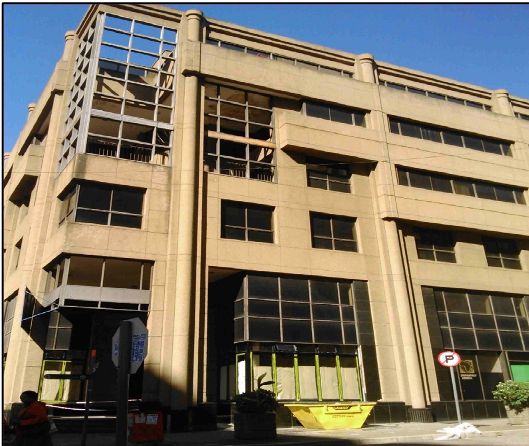
Figure 73: Vacant building along Fox Street (Source: Author's Own)
