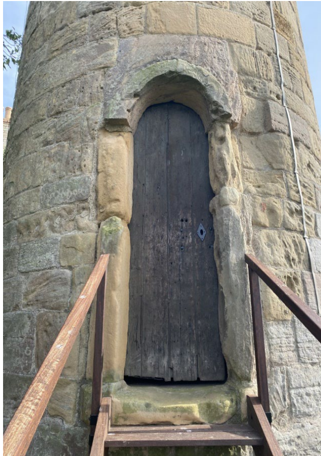
Figure 16. Image of the detail of the elongated doorway showing both the yellow and grey sandstone. Author: Victoria McCormack, 2021.
