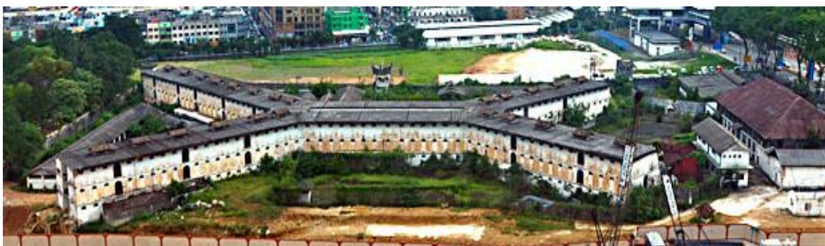
Figure 50 – A photo of Pudu Gaol before its demolition in 2011.
