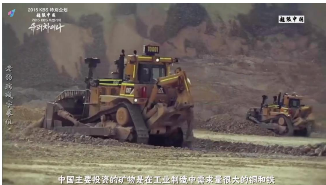
(Fig.7 The excavator is working in Toromocho mines)
