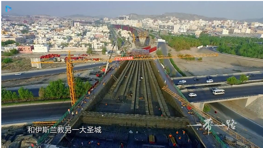
(Fig.20 The construction site of Haramain high-speed railway in Medina.)
