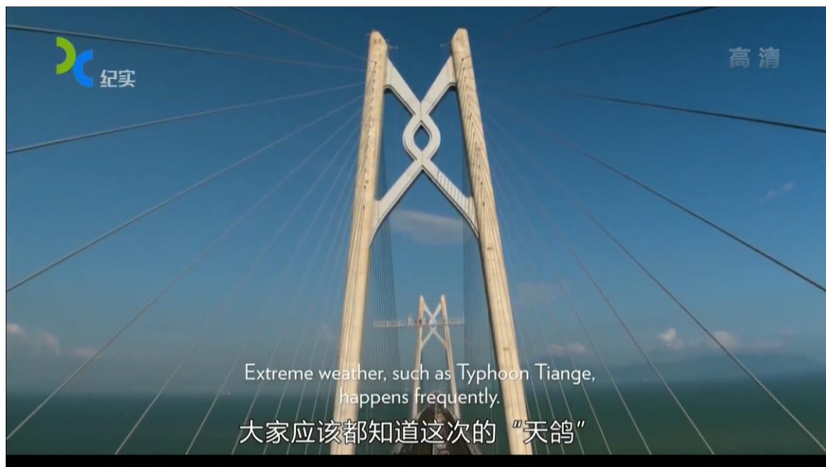
(Fig.41 The drone flies and tilts up to capture the girders and cables. Panning up shot)
