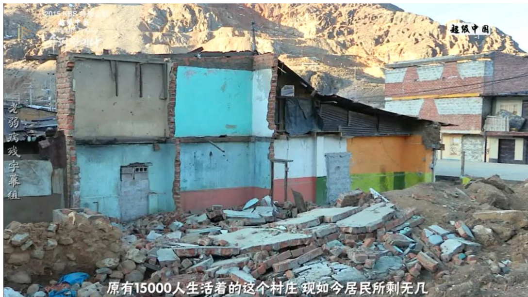
(Fig.10 The broken brick houses in Toromocho)
