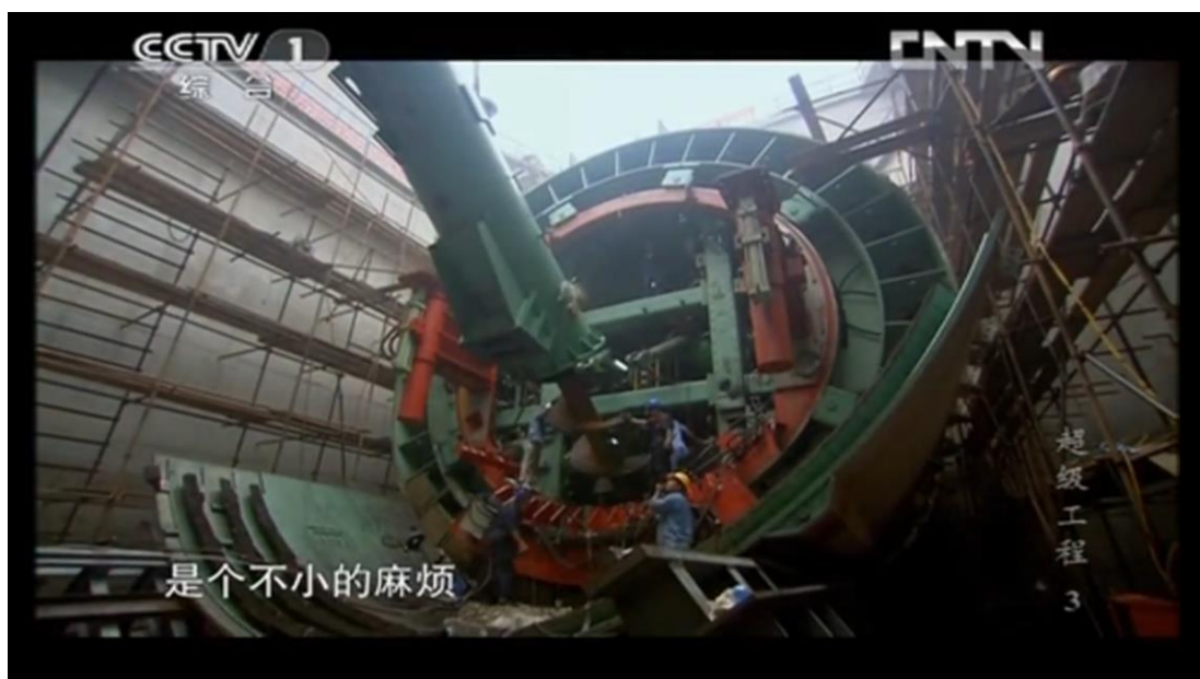
(Fig.5 Tube workers are transferring the sections of a huge TBM to the underground.)
