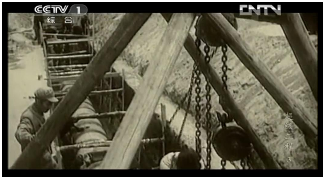
(Fig.2 Chinese workers participate in railway construction with manpower in 1960)
