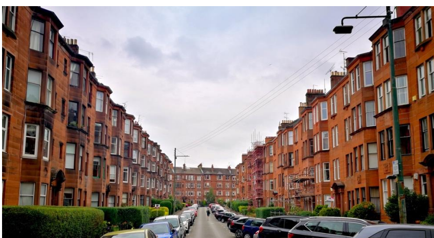
Figure 7.1 Glasgow's tenemental streets generate the feel and ambience of the city - an example of the interplay between the city's tangible and intangible components
