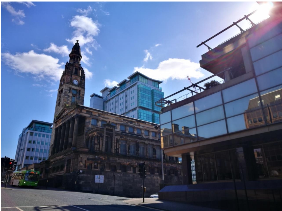
Figure 8.11 Alexander ‘Greek’ Thomson’s St Vincent Street Church | an example of international styles hybridised and embedded in the city to form part of its urban character
