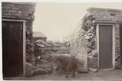
Broken-down Ash-pit, 9c.
