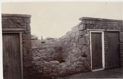
Broken-down Ash-pit, 9c.
