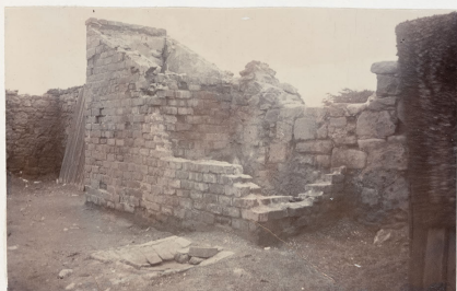
Broken-down Ash-pit, &c.
