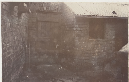
View of a Back-yard: (Tap over sink; ash-pit & privy; dog-kennel, &c).
