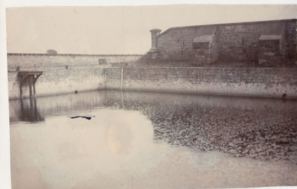
Open & covered Reservoirs.
