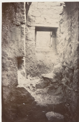
Broken-down Ash-pit, in very close connection with a dwelling.
