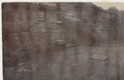
Sewer ventilator & man-hole in a frequent lane.
