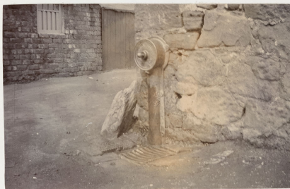
Water-tap: Grating used as a Slop-sink.
