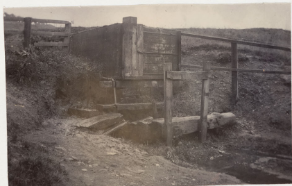
"Old Matt's" water-tank: till 1898.
