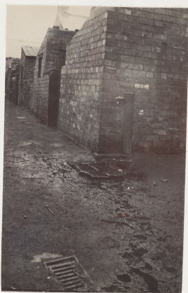
Water-tap: grating used as a slop-sink.
