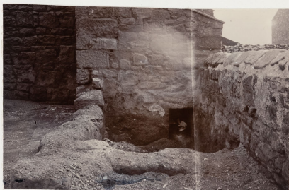
Filthy Ash-pit & Privy.
