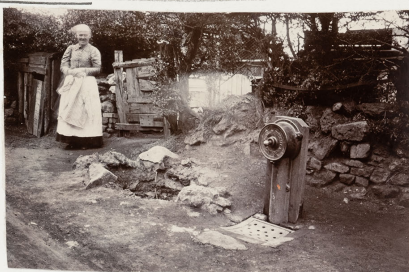
Slop-sink! and Water-tap.
