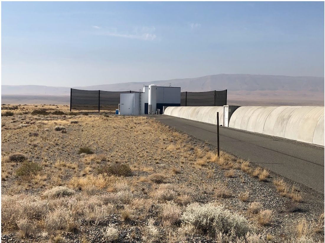
Figure A.1: The wind fence at one of the end stations at LIGO Hanford. Photo credit: Corey Gray
