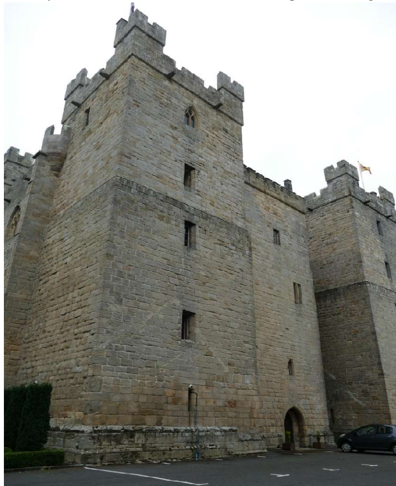
Figure 70 Langley Castle, East Side, site of original entrance. Photo - OB Goulet, 2018.
