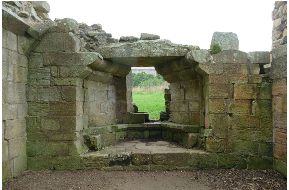
Figure 79 Interior ground floor window, Edlingham Castle (Photo: O.B. Goulet-Paterson, 2018)
