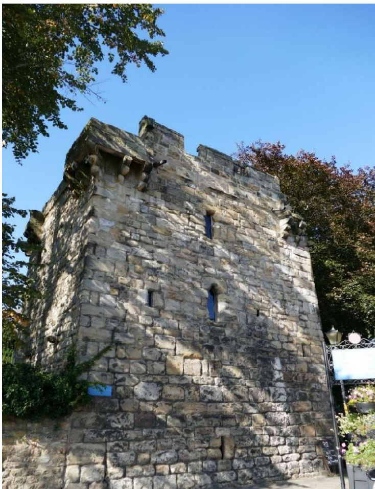
Figure 78 Corbridge Vicar's Pele, as shown from the south, small slit window on ground level and only marginally larger windows on the upper levels. (Photo: O.B. Goulet-Paterson, 2018)
