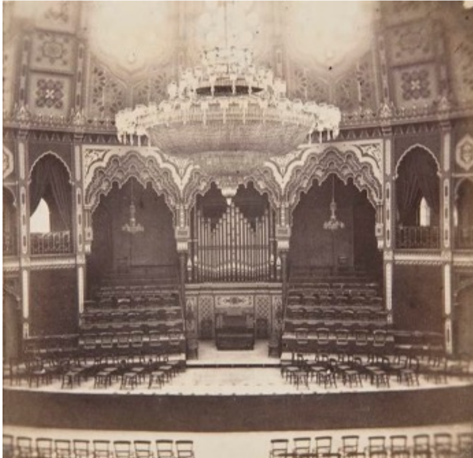
4-6. Photograph showing the interior of “The Dome” at Brighton Pavilion, ca. 1866, monochrome print, H. 86 cm, © The Regency Society James Gray Collection
