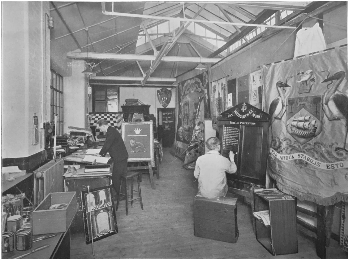
Figure 3.17 View from Kenning's Eagle Wharf Road top floor studio. (Image © G. S. Kenning, 1932, p. 15)
