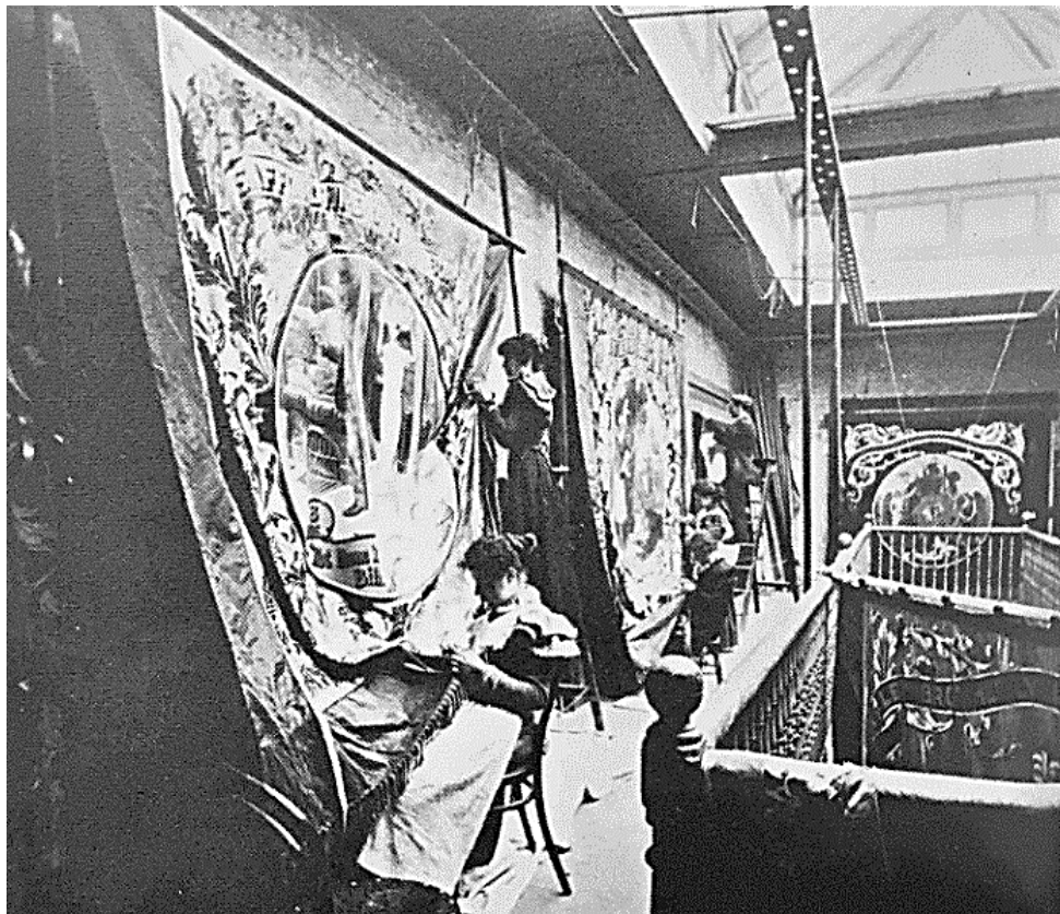
Figure 3.19 View of Tutill's top floor studio in 1899. (Image © Lillingston, 1899, p. 324).
