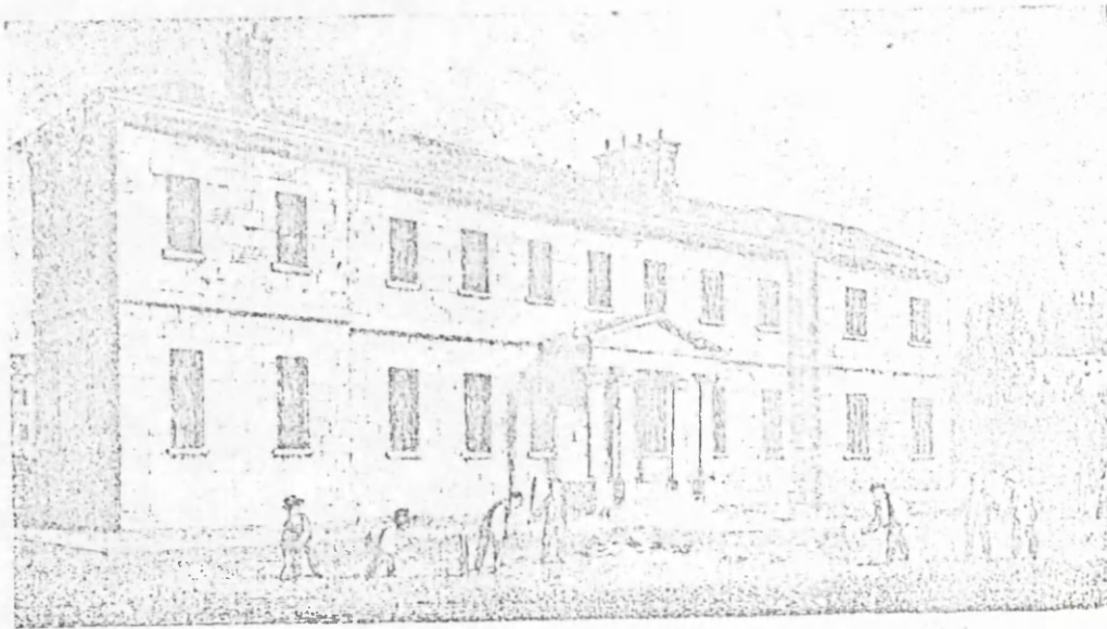
The School at High School Yards, 1777-1929
