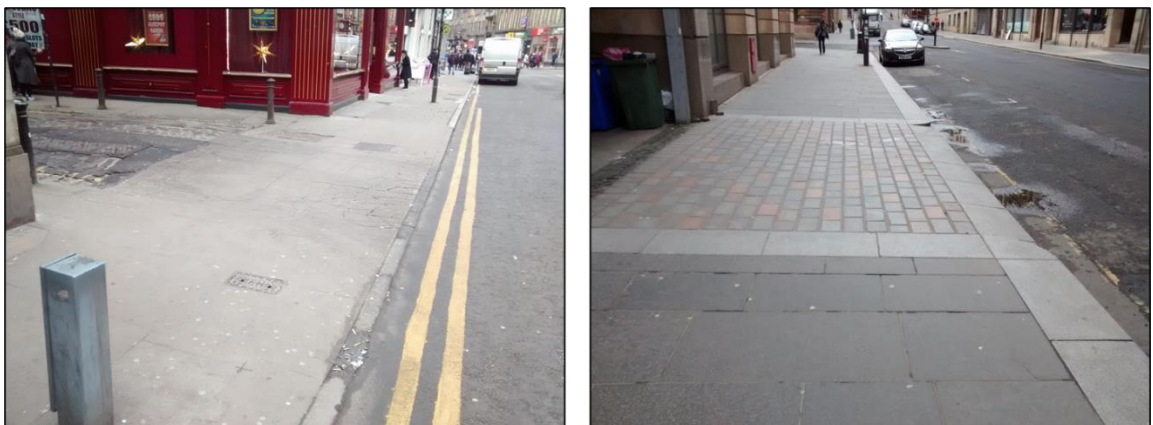
Figure 42: Examples of 1980s continuous footway in Glasgow. The version on the left is more basic but has continuous paving and a narrow junction. The version on the right uses more expensive materials but has a short, steep ramp to clearly signal pedestrian priority. Images © Robert Weetman. Permission to reproduce this image has been granted by Robert Weetman
