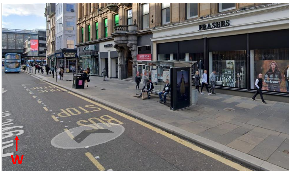
Figure 79: Pinch point control site 1 on Argyle Street where the footway is obstructed by the bus shelter forcing people to walk behind, in front or into the carriageway. Photo © Google Maps.
