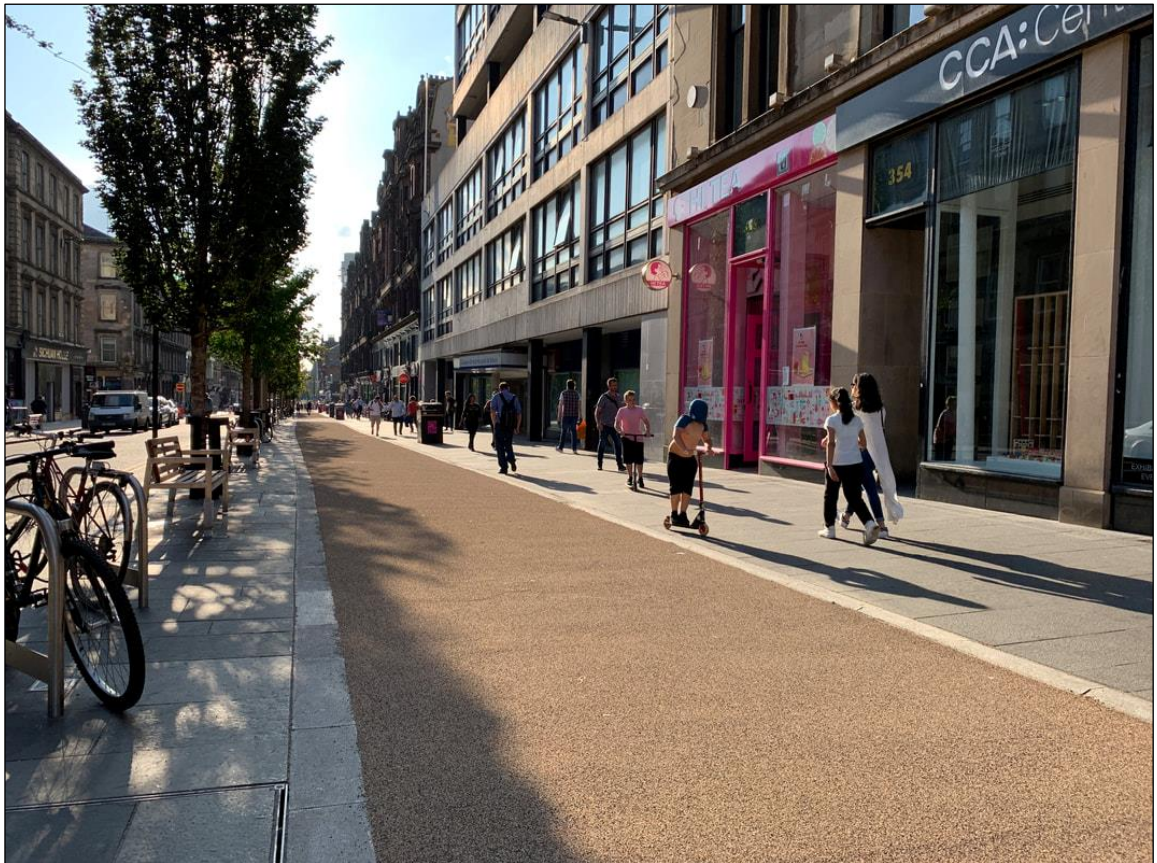
Figure 40: Sauchiehall Street after the Avenues Programme showing widened footway, bi-directional cycle track (prior to painted lines) and furniture zone with benches, trees and cycle parking. Image © Urban Movement Ltd. Reproduced with permission.
