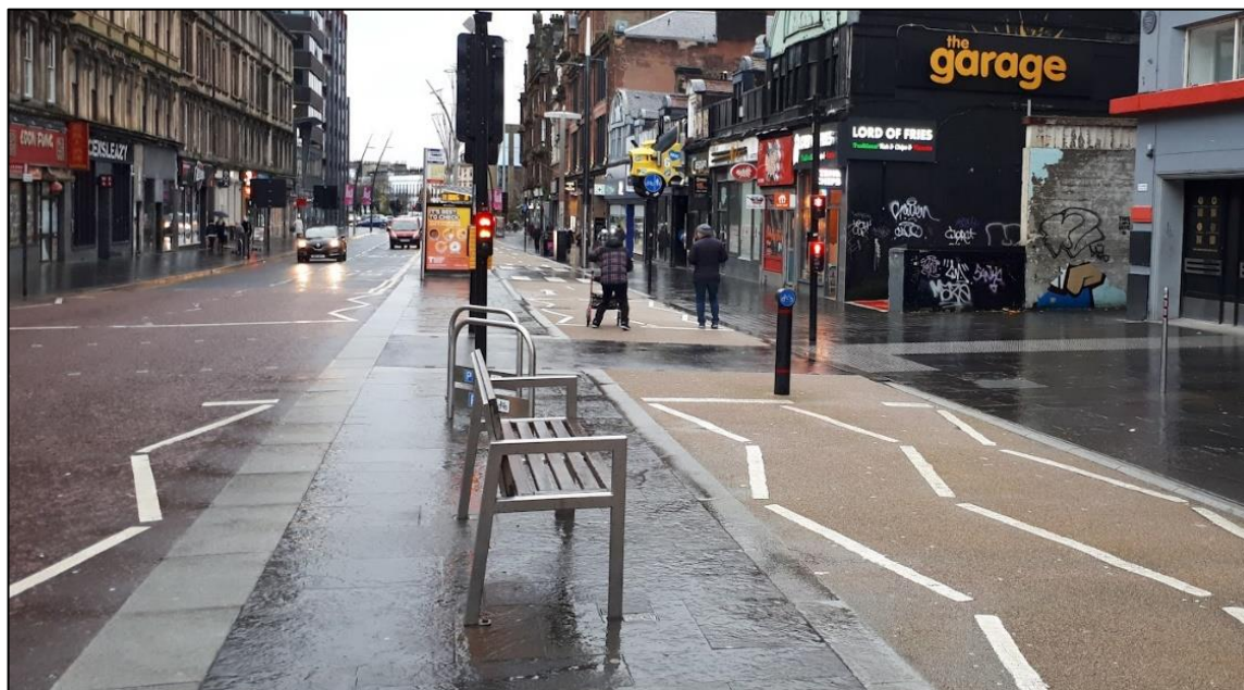
Figure 57: Benches installed at regular intervals in the central median along the length of the new section of Sauchiehall Street. These are wooden with backs and armrests, oriented such that they face the street with their backs to the carriageway directly behind. Image © author.
