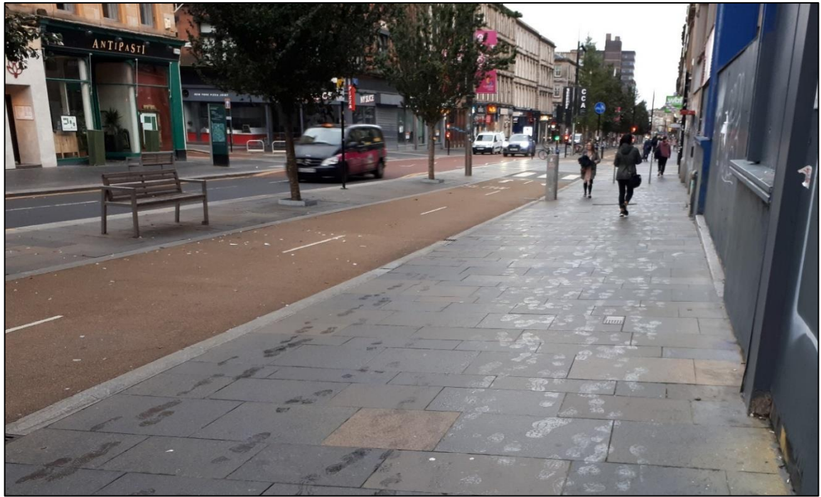
Figure 17: Footway-level cycle track adjacent to widened footway in the regenerated section of Sauchiehall Street. Photo © author.
