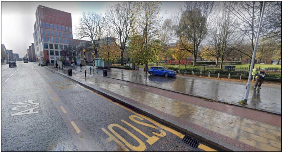
Figure 6: Oxford Road, Manchester. This busy transport corridor is a key route in the 'Bee Network'. It was re-profiled to introduce segregated cycle tracks (red tarmac) and widened footway. Image © Google Images.
