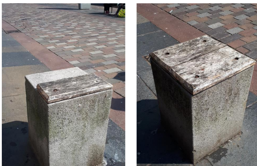
Figure 101: Example of the stone posts on Argyle Street, which were being used as informal seating. Some have been retrofitted with wooden slats on the top, presumably to make them more comfortable to sit on, although these slats were sometimes missing in part or entirely. Images © author.
