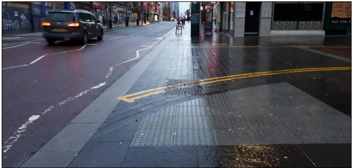
Figure 93: Pitt Street side road is designed such that the footway is flush with the carriageway, providing no physical deterrent to drivers to stop them cutting the corner when turning in. Image © author.
