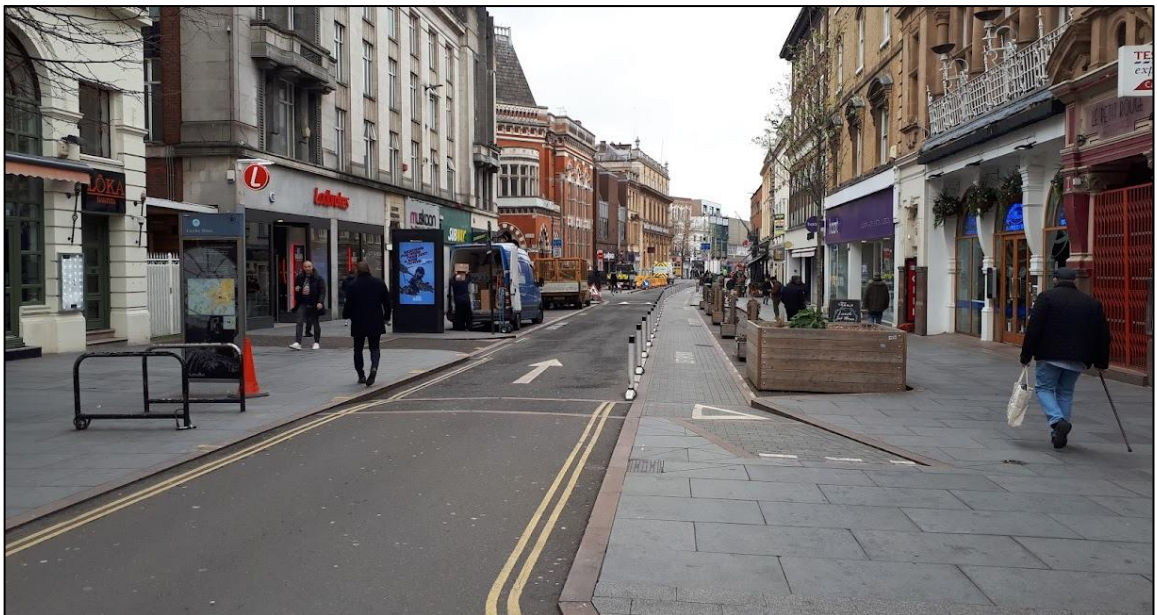
Figure 7: Granby Street, Leicester. This street was one of several regenerated as part of the Connecting Leicester programme, which aimed to regenerate a network of streets across the city. It introduced contraflow cycling in the carriageway, widened footway and reduced vehicle dominance. Image © author.
