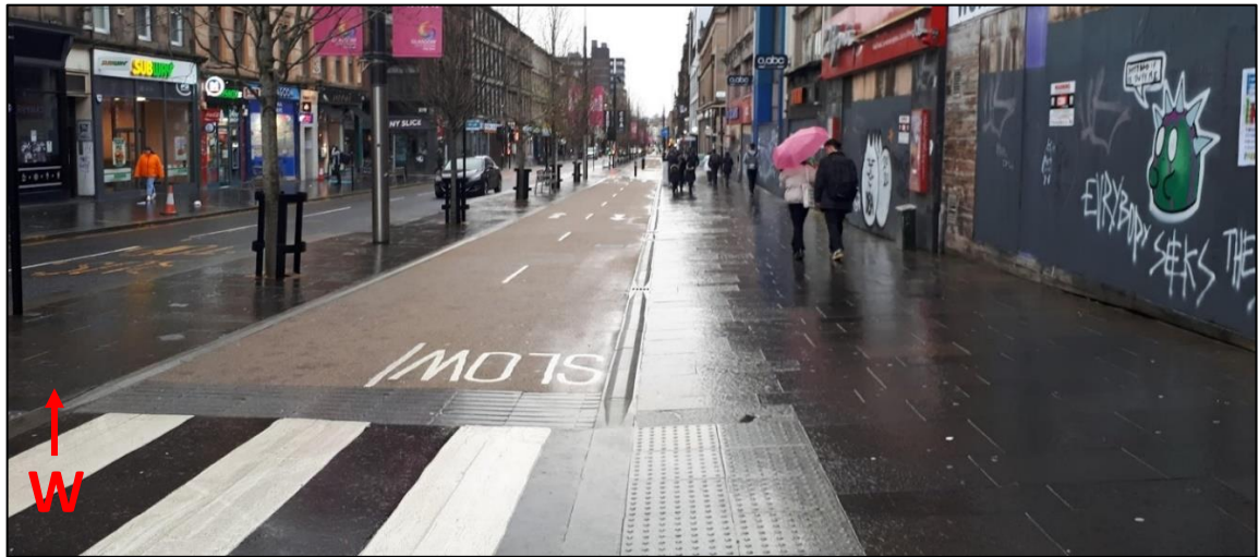
Figure 76: Footway-level cycle track on the north side of Sauchiehall Street showing footway and bi-directional cycle track, with a 'mini' zebra crossing and tactile paving over the cycle track. Note the raised delineator kerb between the footway and cycle track, designed so someone using a long cane can theoretically detect the edge of the cycle track. Image © author.
