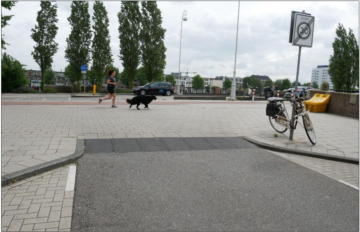
Figure 46: Example of short, steep ramp used with continuous footway in the Netherlands. Image © Robert Weetman. Permission to reproduce this image has been granted by Robert Weetman
