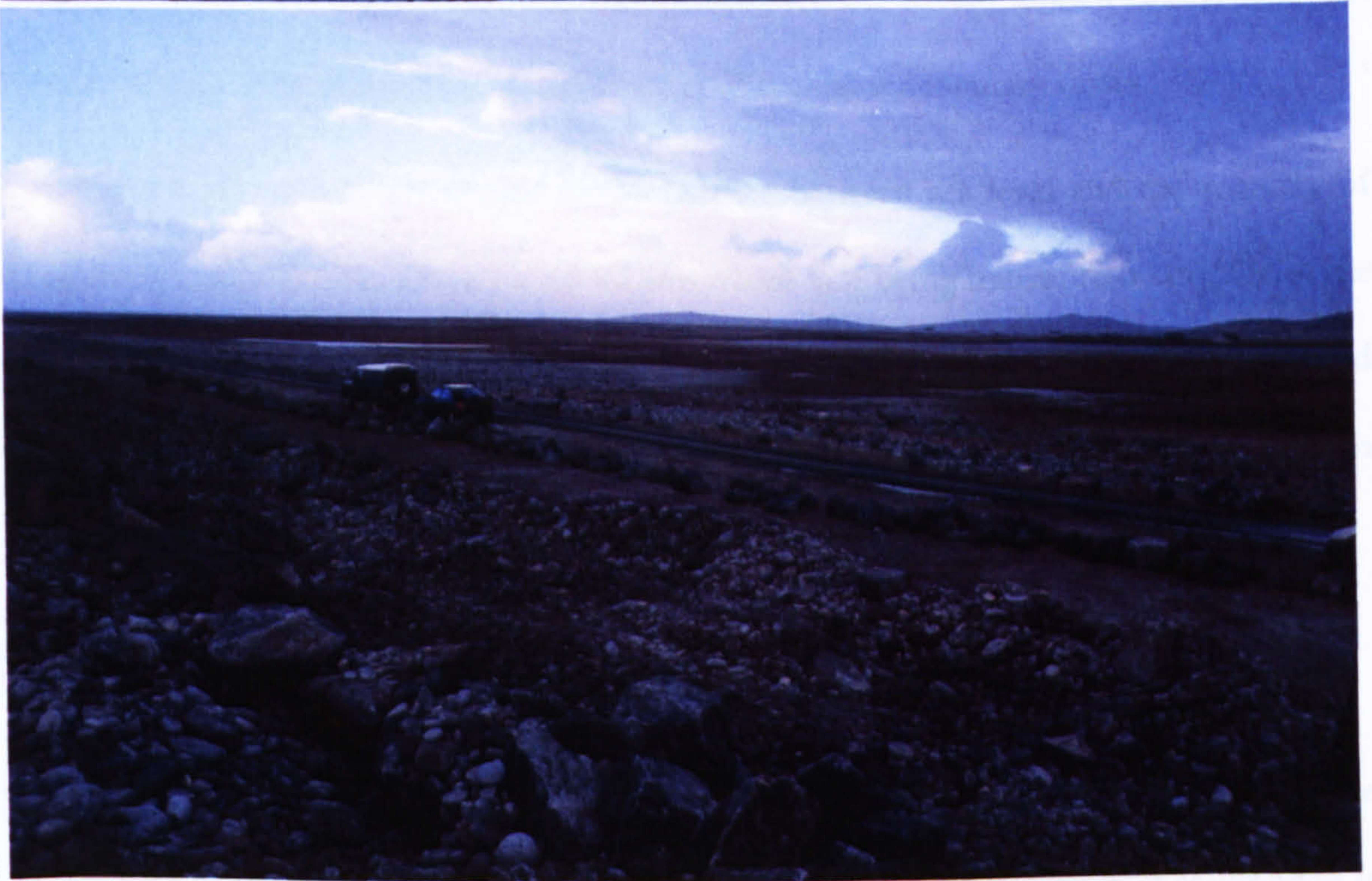
Figure 2.16 Storm damage as the gravel barrier rolls over a road at Stoneybridge, South Uists. A, from the air, B from the top of the ‘repaired’ gravel ridge.
