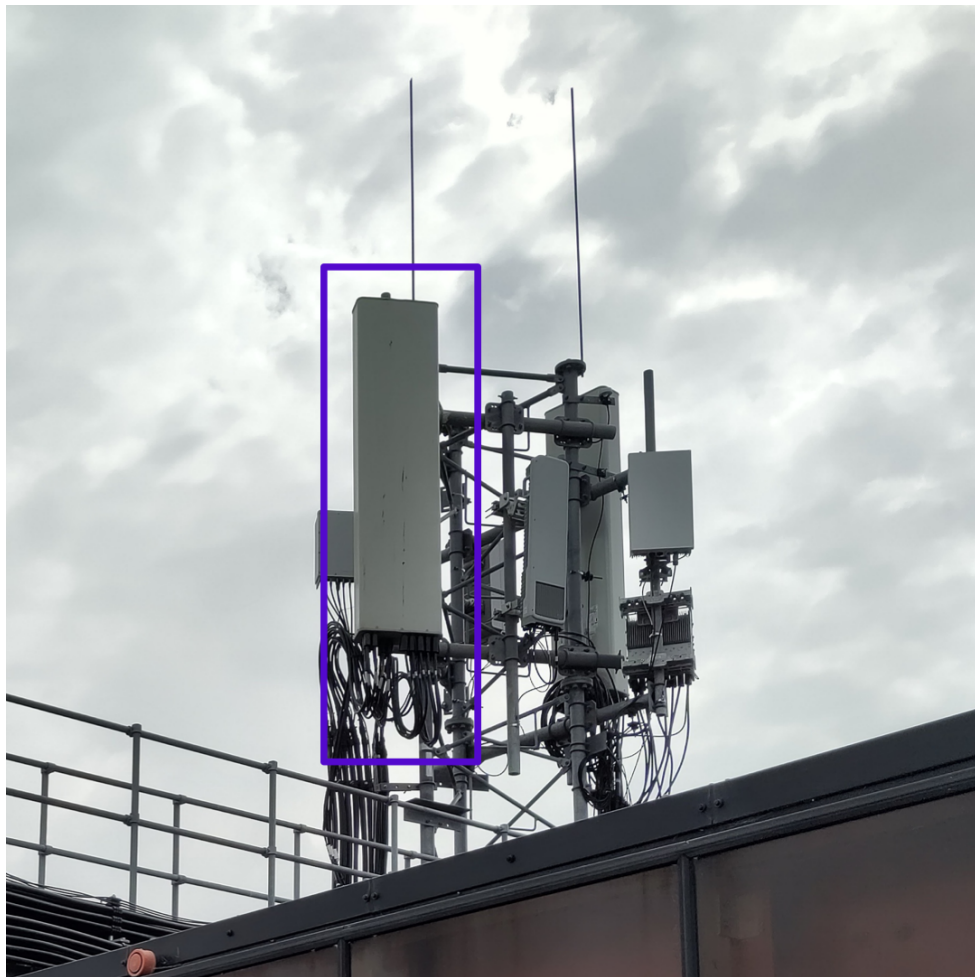
Figure 5.8: Sector antenna used in the measurements. The antenna points north, with 90^\circ and 6.5^\circ beamwidths in azimuth and elevation, respectively.
