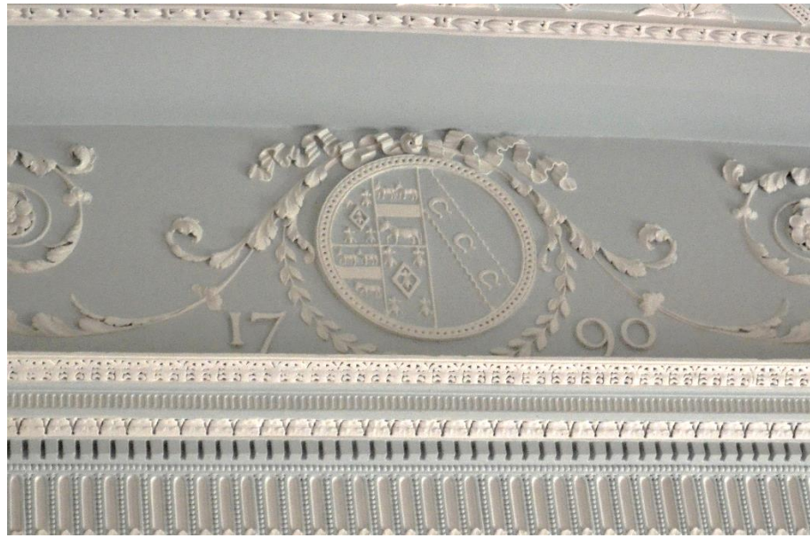
Ceiling Detail, Drawing Room, Georgian wing, Farnley Hall, June 2023 (Author's photograph)
