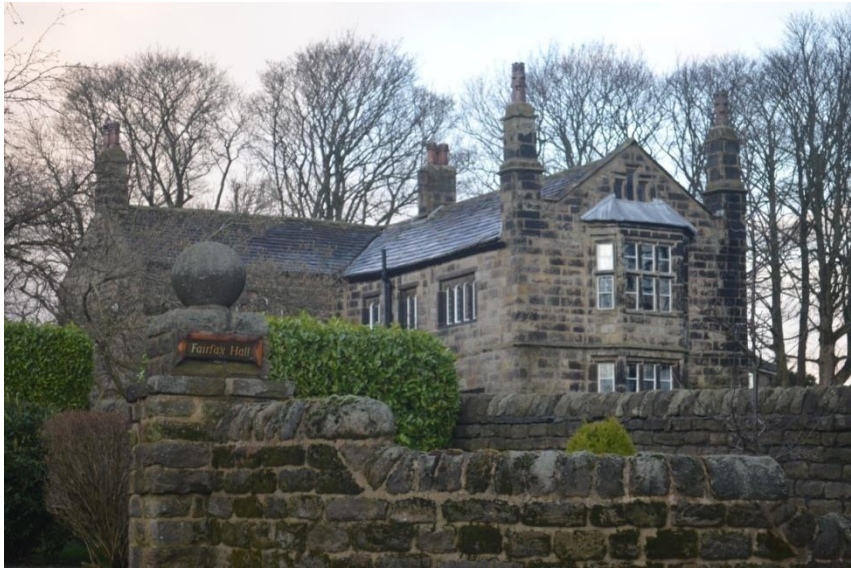
Fairfax Hall, Menston, February 2020 (Author's photograph)
