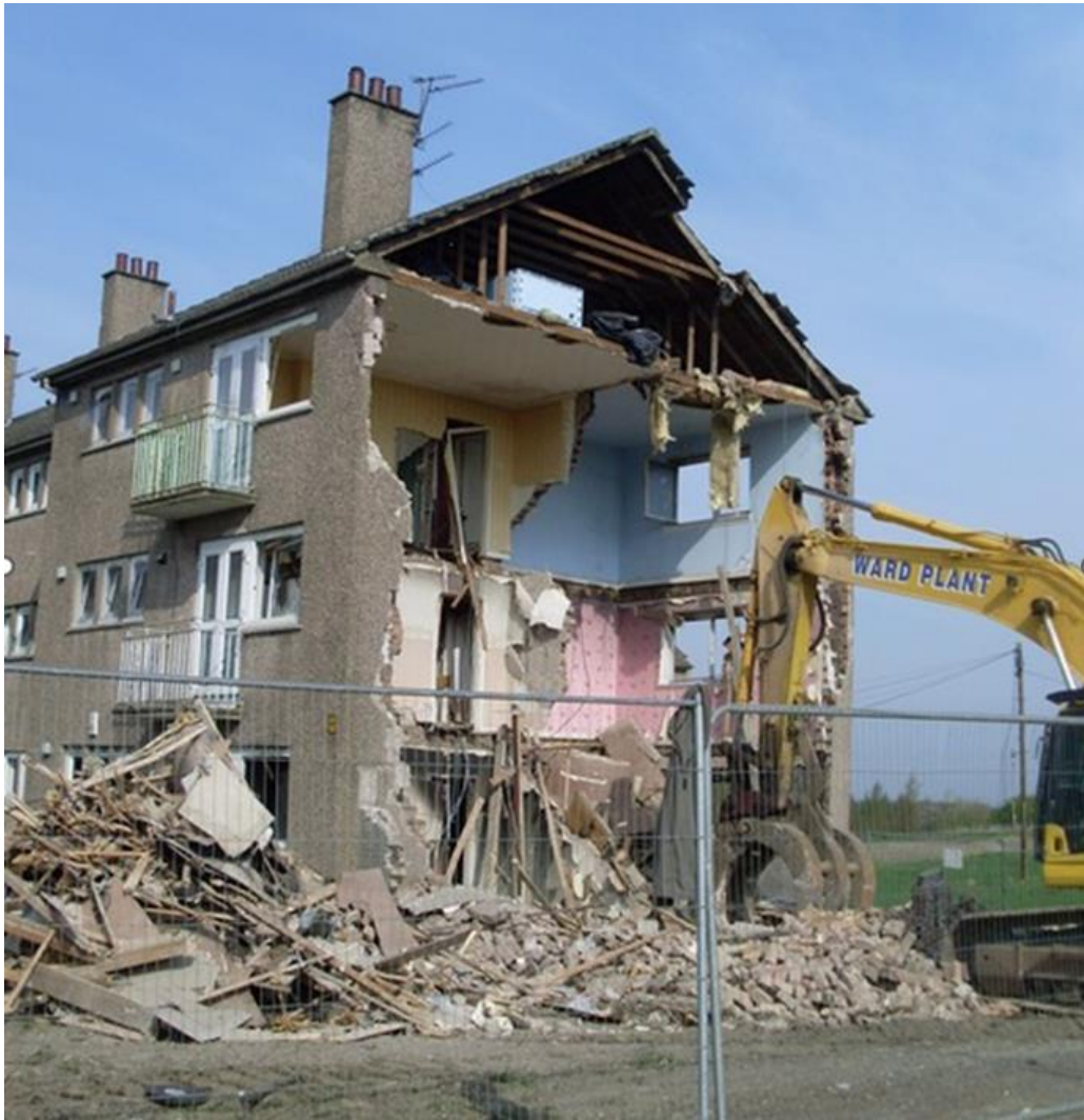
Figure 4.10 Demolition of Council Housing near Lochwood, Easterhouse, 2003
