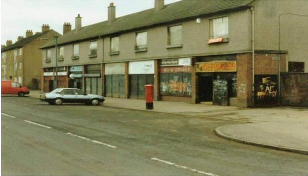
Figure 4.12 Provan, Easterhouse, 1980s
