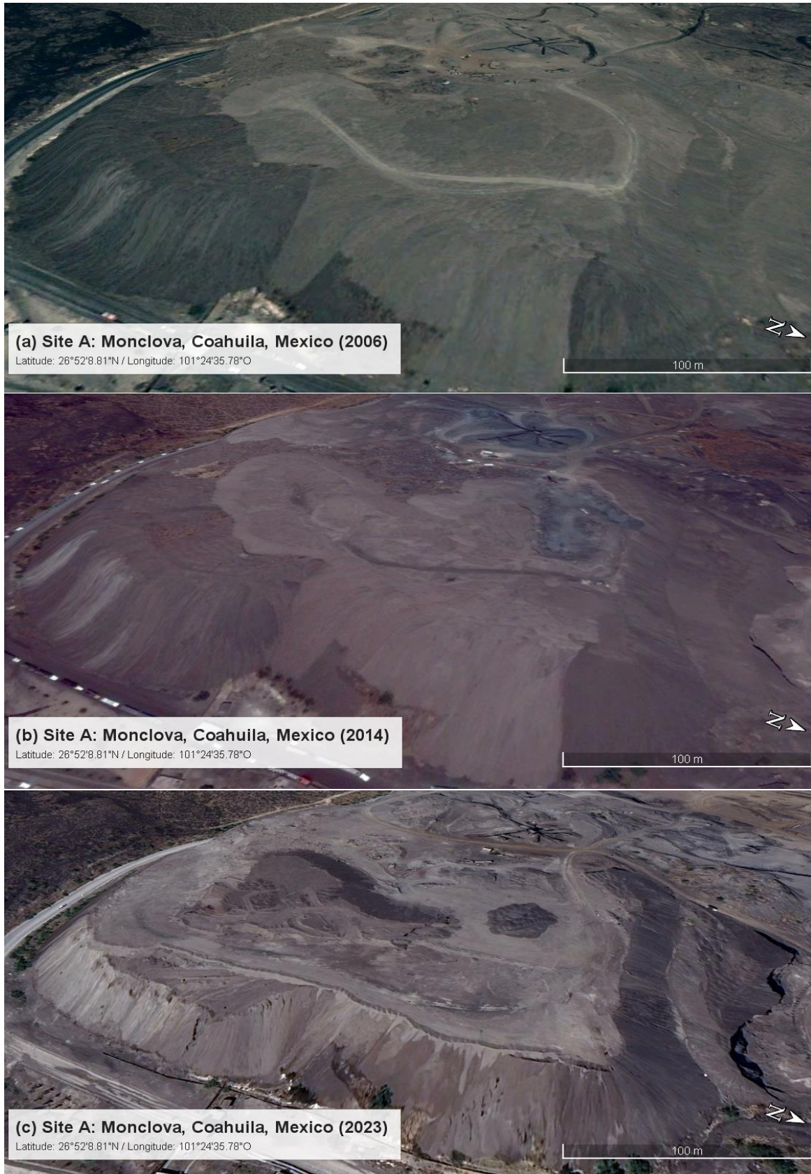
Figure 16 View of slag heap Monclova, Mexico across time: (a) 2006, (b) 2014, (c) 2023; images from Google Earth Pro (2024).
