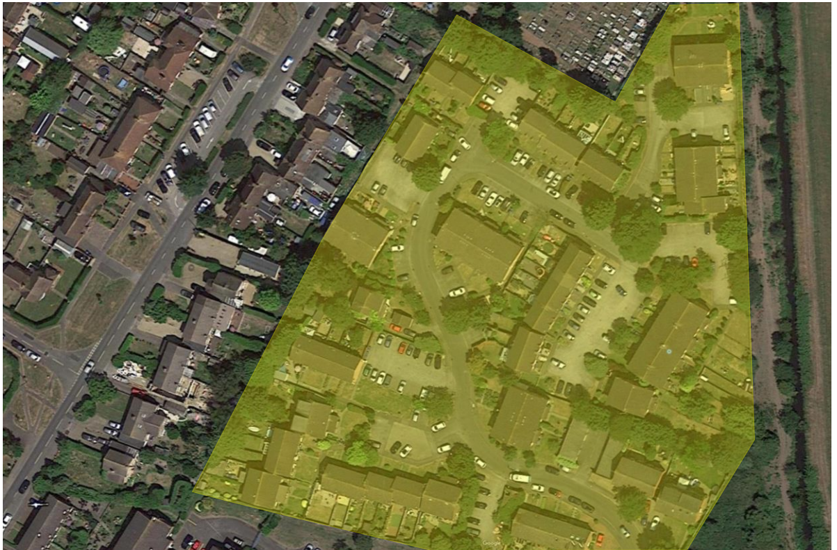
Figure 3.1.1.1: Satellite view showing the 1980s addition to Road A highlighted in yellow (Google, 2020).
