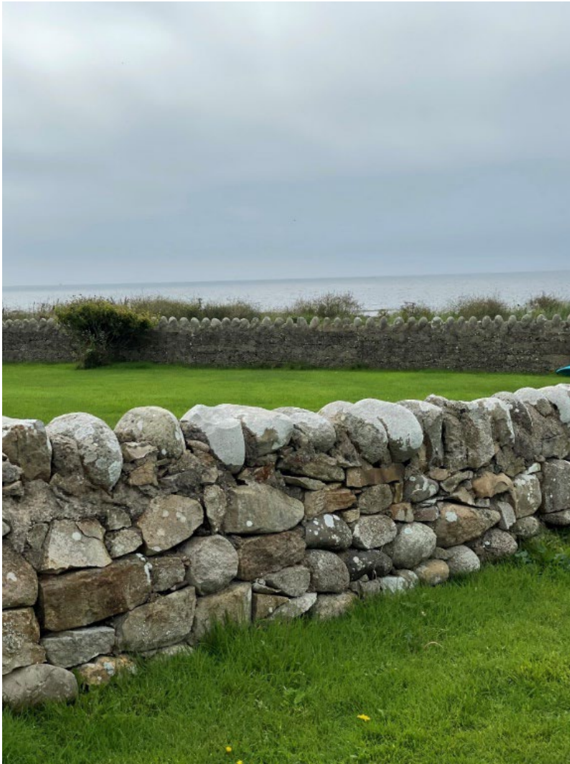
Figure 88: One of many Blackwaterfoot walls of roughly this period that likely reused cairn material
