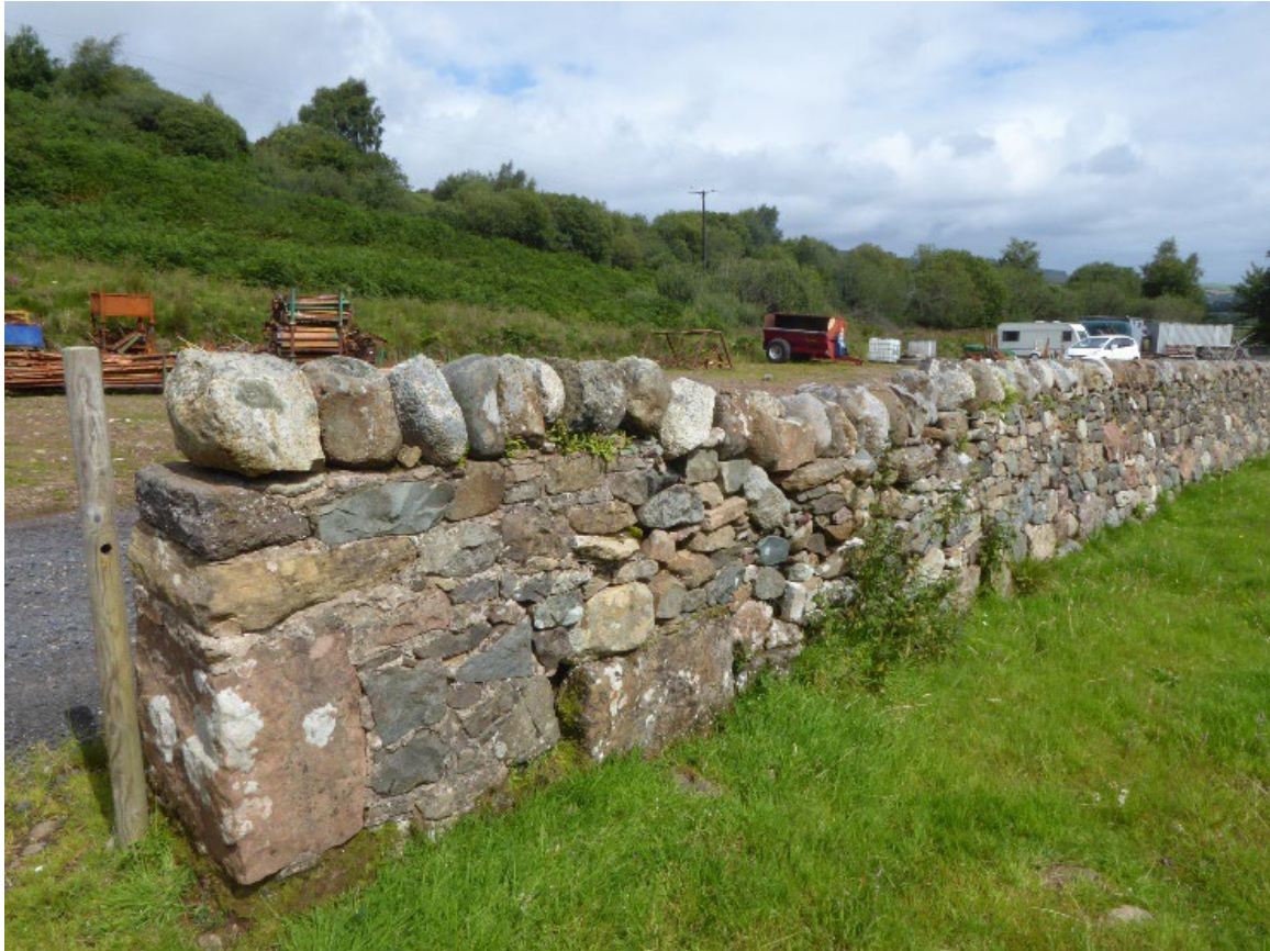
Figure 84: Small part of the wall at Monamore.
