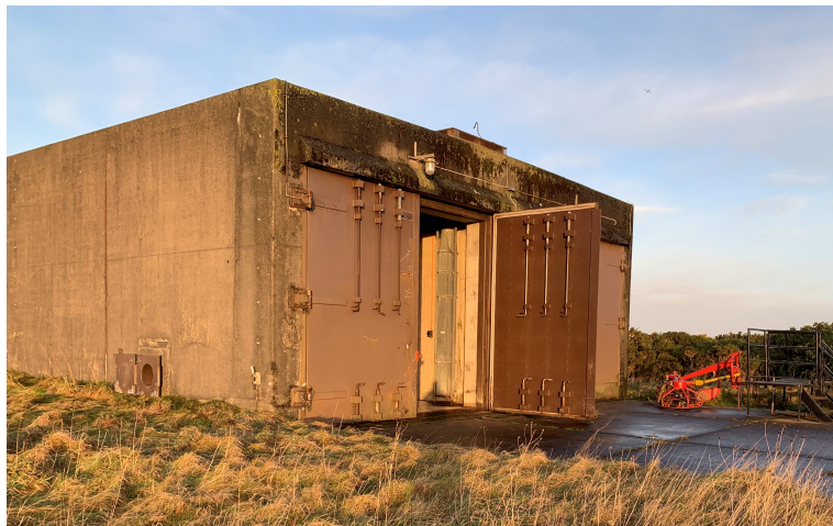
Fig. 4.1 076 Refueling Vehicle Shelter (RVS) used as a temporary propulsion test facility.
