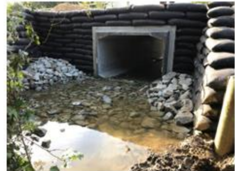
Culvert headwall at installation, June 2021
