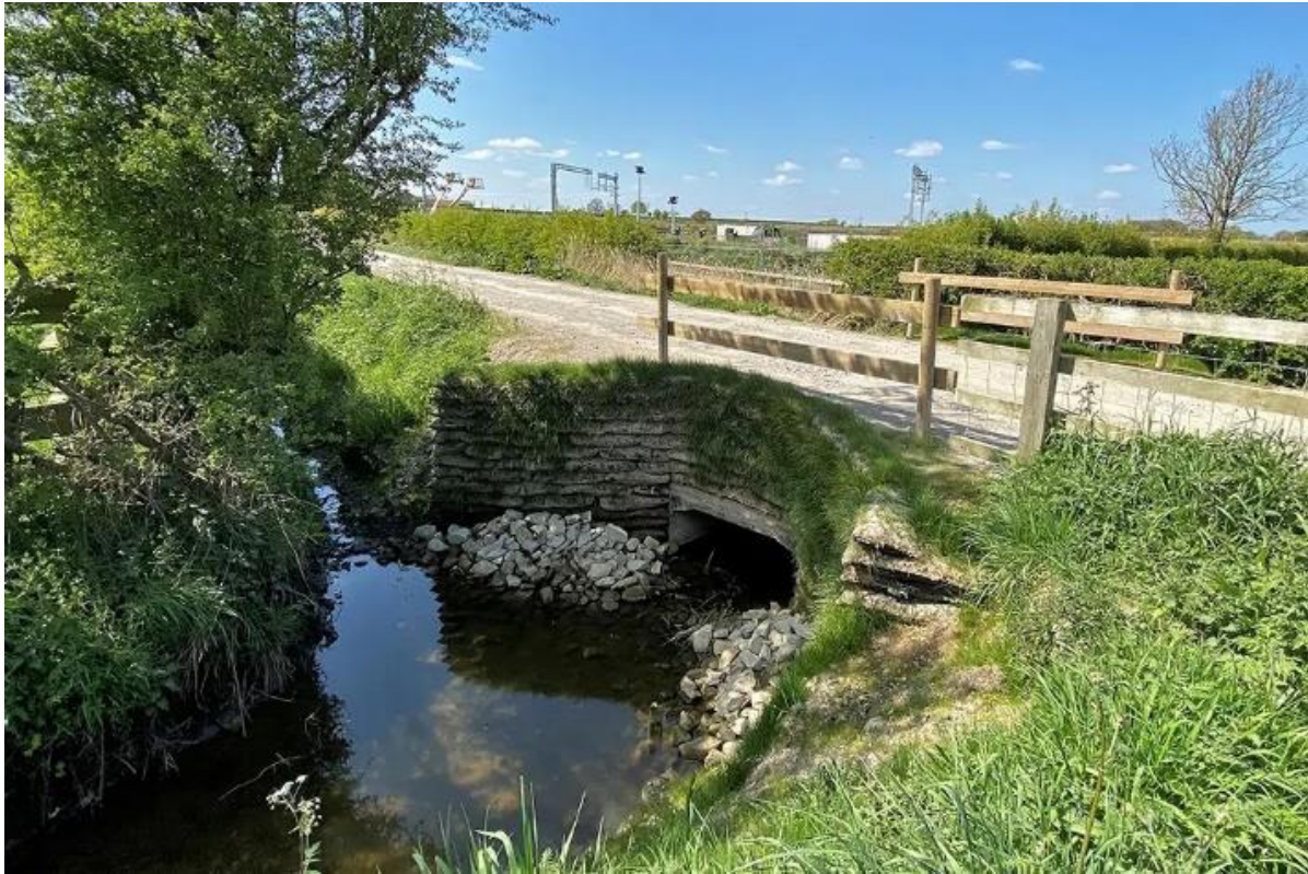
Figure 5-3 Vegetated culvert headwall adjacent to railway at Brumber Hill, Yorkshire
