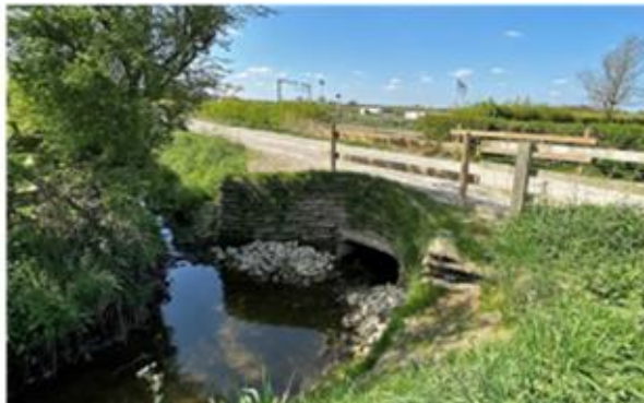
Vegetation established on culvert headwall, 2023
