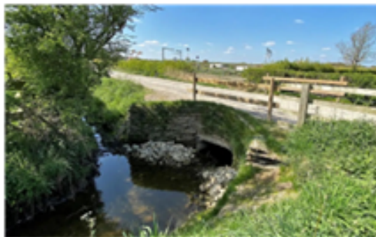
Vegetated headwall culvert, Brumber Hill, UK (Photo credit: Scott Parnell Ltd., 2022)
