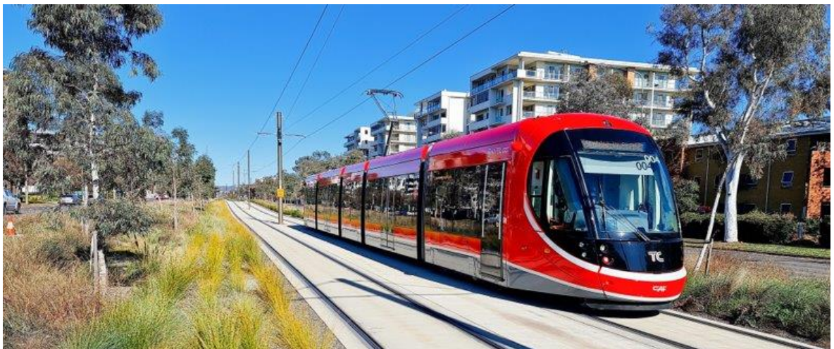
Figure 1-3 Sustainable drainage system adjacent to the track on Canberra Light Rail, Australia (Source: Blackwood, 2023)
