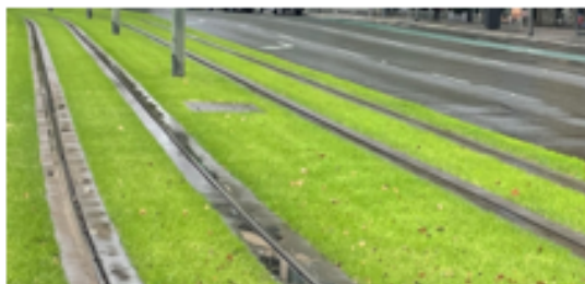
Green track at Victoria Square, Adelaide, Australia
