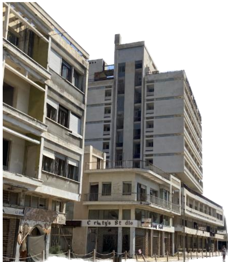
Fig. 14 Abandoned buildings inside Varosha, author's own image, 2023.
